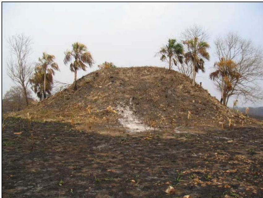
Fig. 3: E1, one of the major monumental buildings in Las Palmitas, covered by sediments and huano palm-trees. The photo was taken in May, soon after the cyclic cremation of the vegetation, a practice the local farmers employ to increase the fertility of the soil. The shape and general aspect of this mound is typical for most of the local Maya "pyramids" (photo: C. Ardelean).
