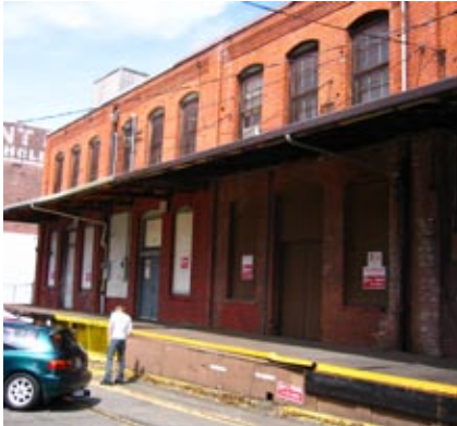
Loading docks on Commerce Street
