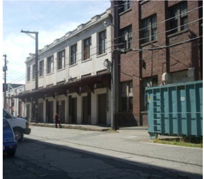
The east side of Commerce Street has some existing sidewalks, loading docks and a de-facto shared use of the street.
