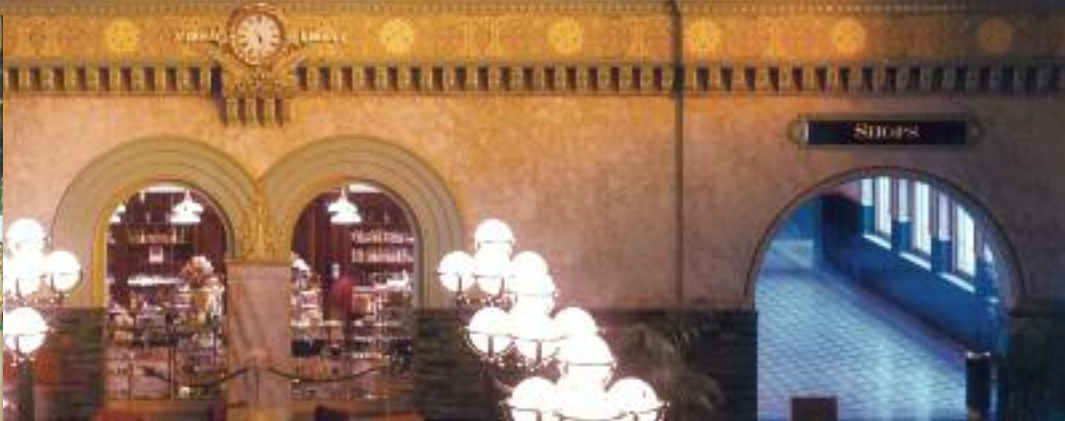
Opposite and top: The decorative painting and plaster restoration at St. Louis Union Station (built 1894) reflects a portion of one of the largest adaptive re-use projects in the U.S. CSS also restored the large Tiffany-style stained glass window over the grand staircase.
