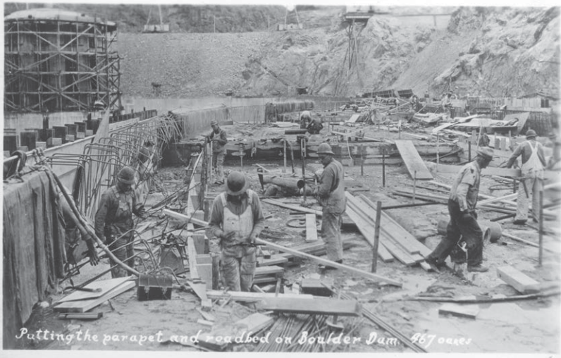
Workers cut and prepare building materials at the Boulder Dam site (1933).
