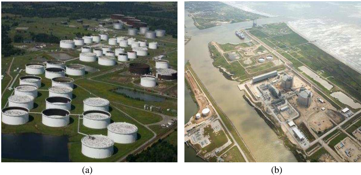
Figure 3: Crude oil and Natural gas tank farm (a) in Cushing, Oklahoma, USA [14] (b) in Brazoria County, Texas, USA[15]
