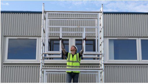
13. Fit 2 Advance Guardrail frames, hooks facing outwards ensuring the top hook is located above the top rung.
