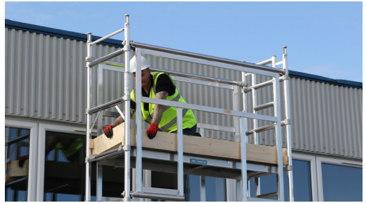
16. Once you have reached the desired working platform height. Correctly fit your Toe-board system as shown.
