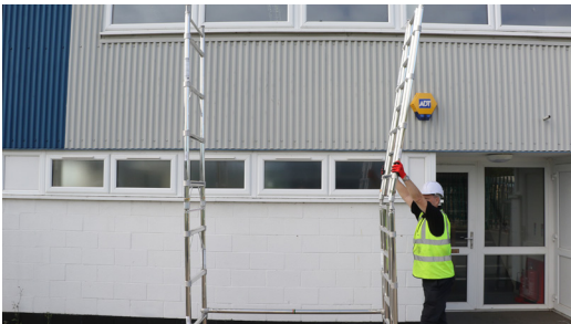
5. Add further frames ensuring the ladder is continuous.
