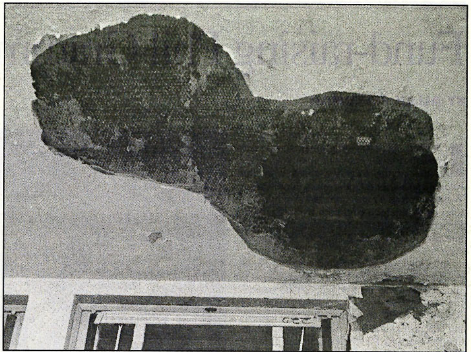
Library ceiling at Brownsville intermediate school, 1986.
