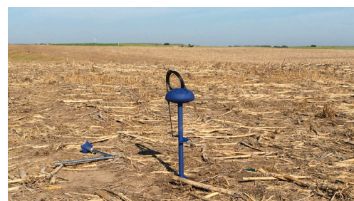
Soil moisture probe being installed
