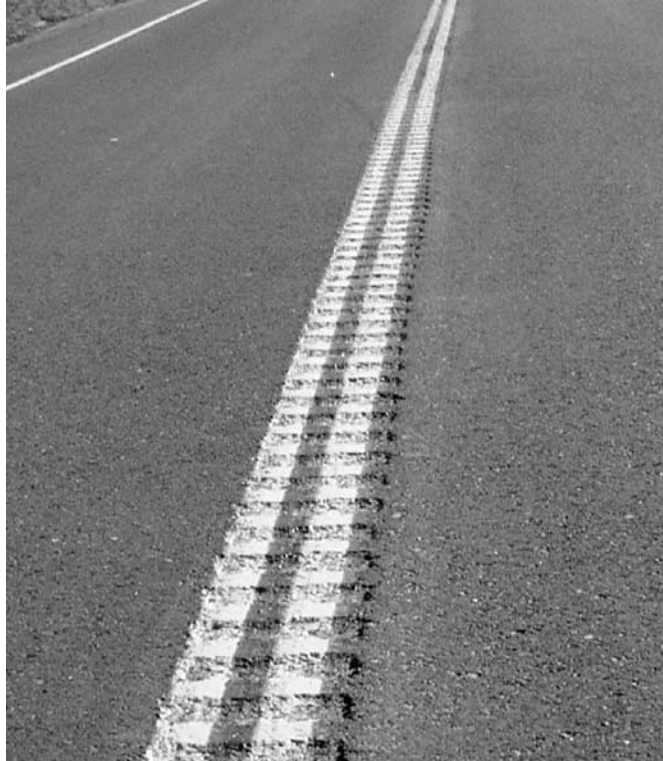
EXHIBIT V-6 Centerline Rumble Strips (Photo Provided by Caltrans)
