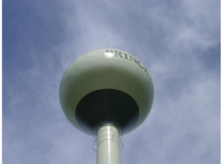
New Elevated Storage Reservoir
