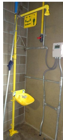
Photographs at a new water treatment plant finished in 2012 of the prototype operations screen, pumps, softeners, and emergency eyewash and safety shower.
