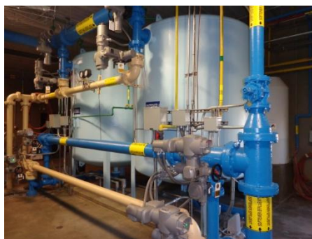
Photographs at a new water treatment plant finished in 2012 of the prototype operations screen, pumps, softeners, and emergency eyewash and safety shower.
