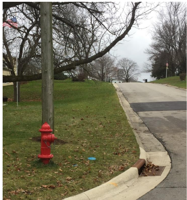
New fire hydrant as part of upgraded distribution system
