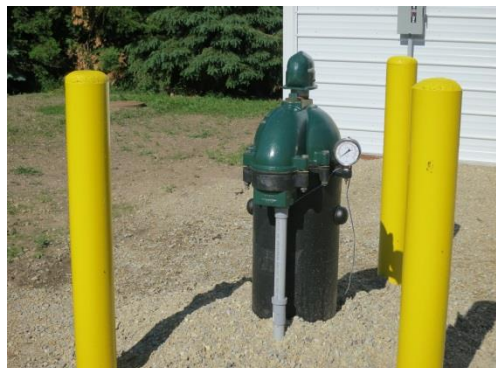
New well with protective posts
