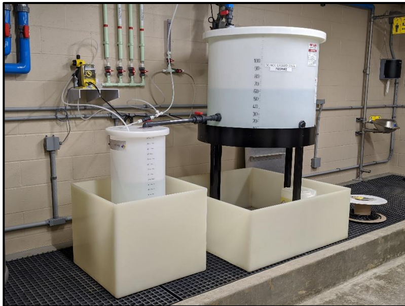
Polyphosphate Feed and Day Tank
