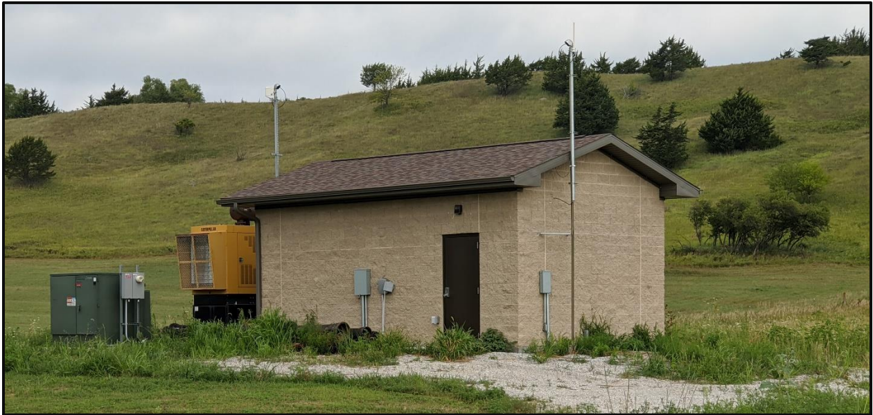
Well house with emergency generator
