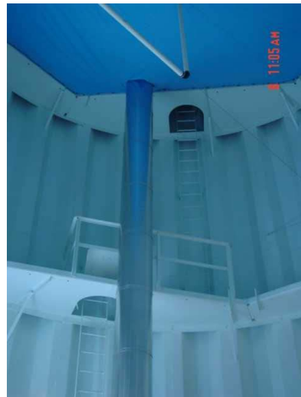
Interior of an elevated water storage tower
