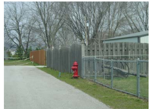
New fire hydrant in the distribution system
