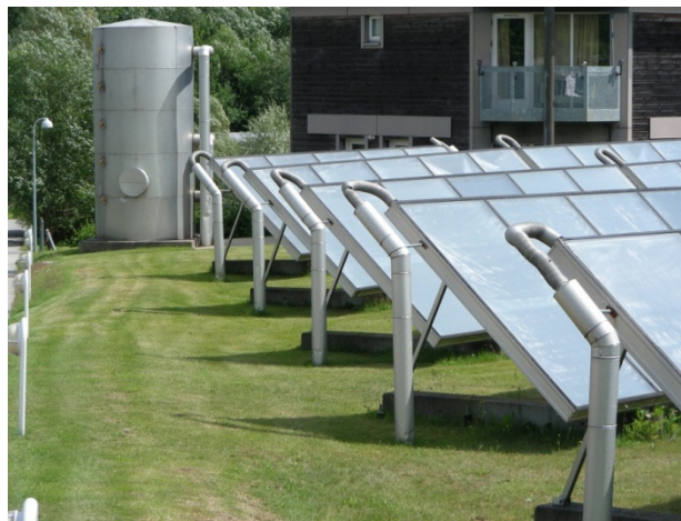
Figure 3: Example of a solar district heating system
