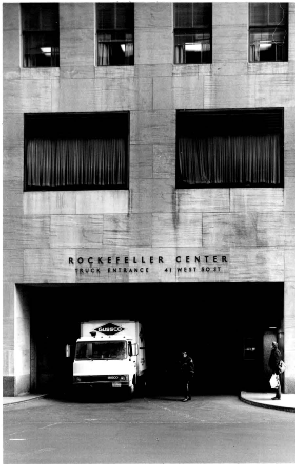
Truck entrance, 41 W. 50th Street.
