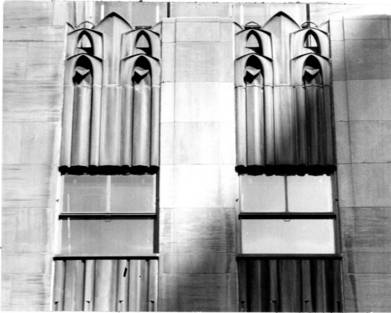
Four-eyelet spandrels, upper setbacks and roof level.
