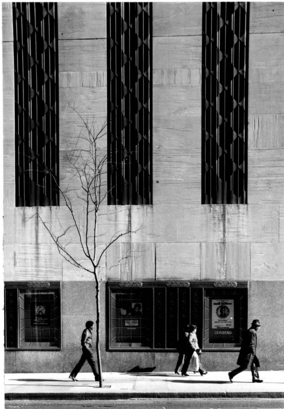
Fire escape screens & display windows, 50th St. facade.
