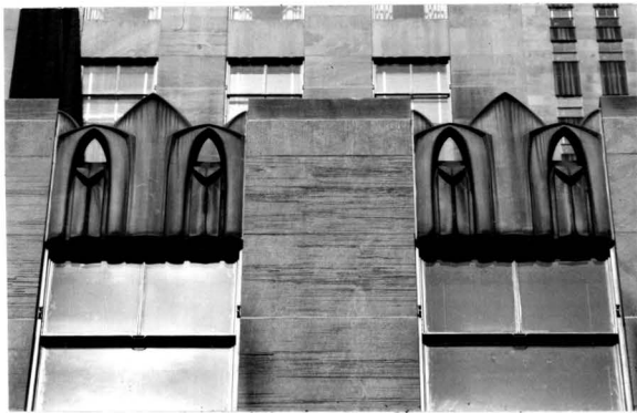
Two-eyelet spandrels, east facade slab setbacks.
