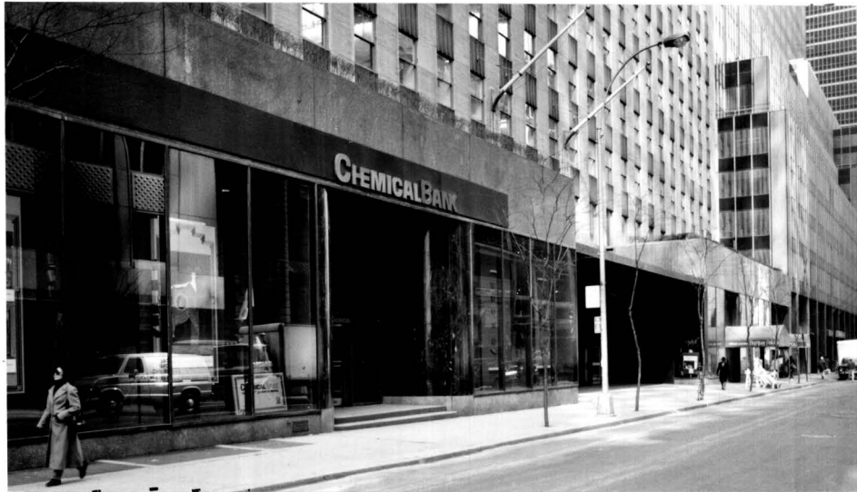
W. 52nd Street elevation, view west.
