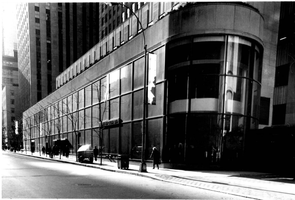
West 49th Street elevation, view east.
