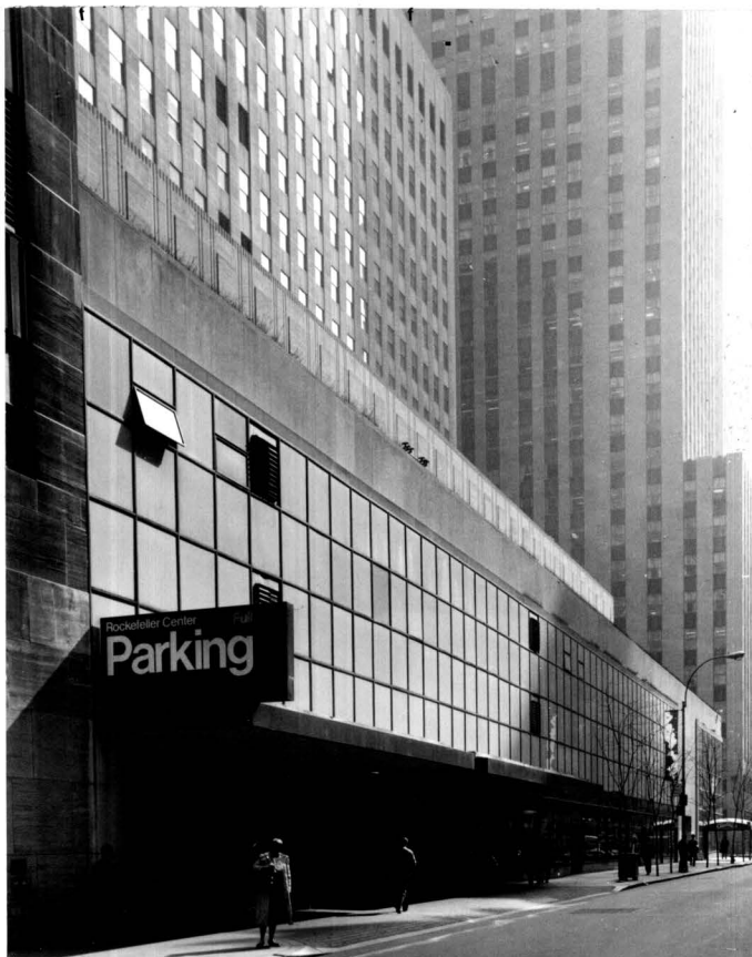
West 48th Street elevation, view east.
