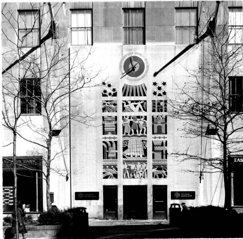
LIMESTONE SCREEN 25 W. 50th St. Entrance Lee Lawrie Installed 1935
