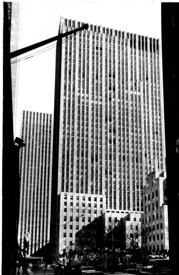
View from southwest; Warner Communications Building at left.
