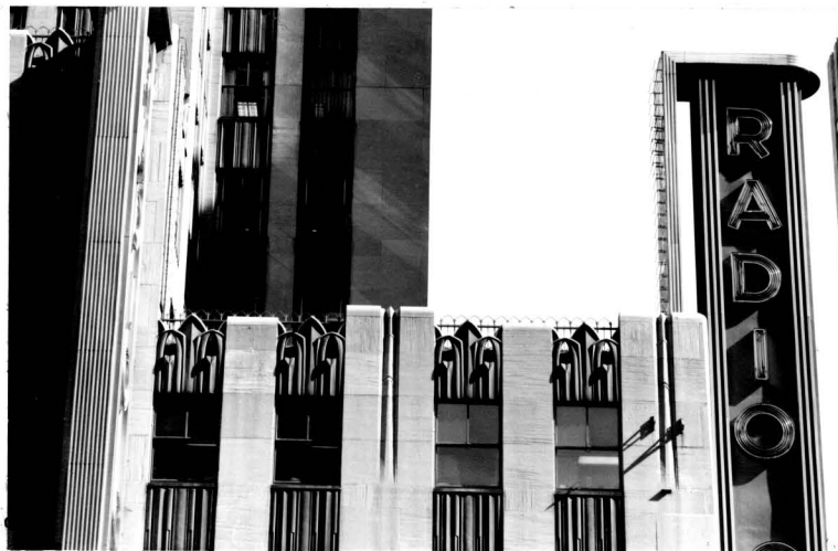
Foliolate spandrels and Gothic arcade, extension over Radio City Music Hall.
