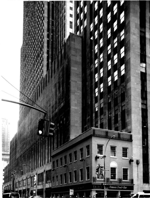
View east along 50th St. Corner property originally uncontrolled. RCA Building West at right; 11-story NBC studios at left, RCA Building slab above.
