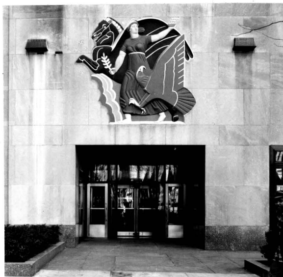
LIMESTONE RELIEF 14 W. 49th St. Entrance Lee Lawrie Installed 1937
