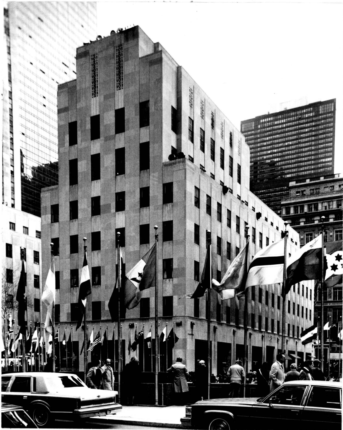
Rear Facade, View East
