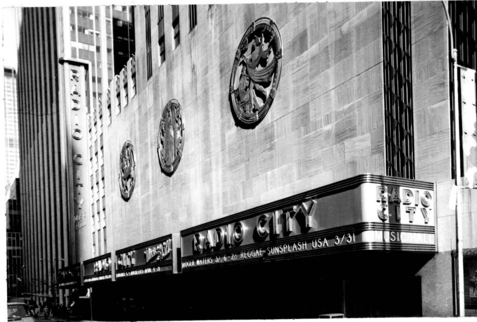
THREE METAL & ENAMEL PLAQUES W. 50th St. Facade (view west) Hildreth Meiere Installed 1932
