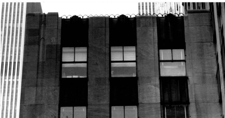
Stepped vertically ridged spandrels, lower setbacks and above NBC studios.
