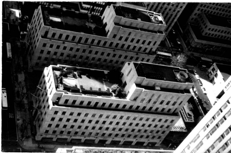
Bird's-eye view from northeast. British Building at center, La Maison Francaise above. International Building, far right.
