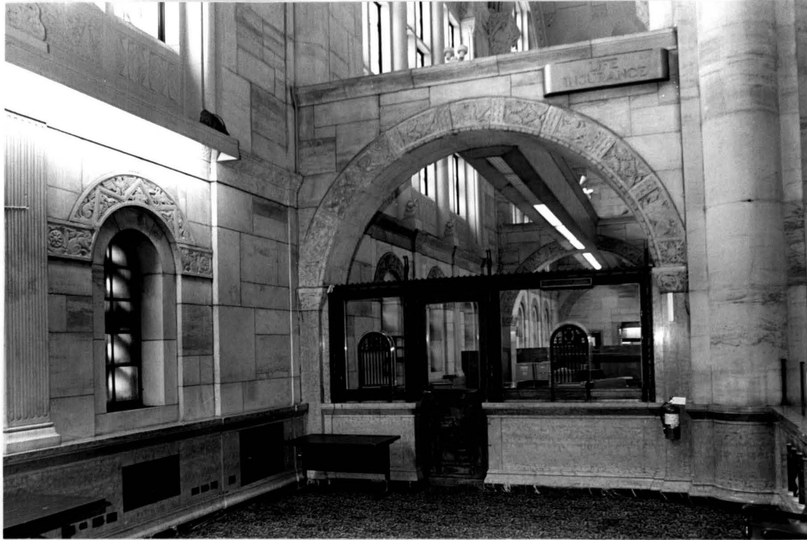
31. Banking room, south bay west aisle (new accounts area) looking north, 1996
