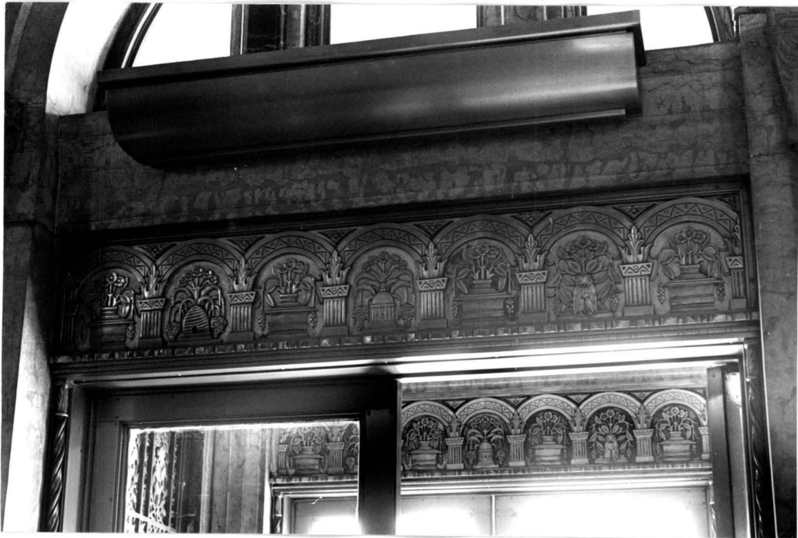
3. Entrance vestibule, spandrel panels above doors, 1996
