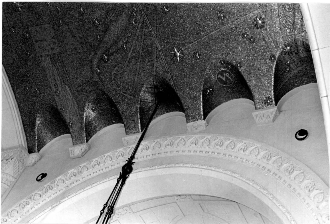
44. Banking room, detail of mosaic vault of nave, 1996
