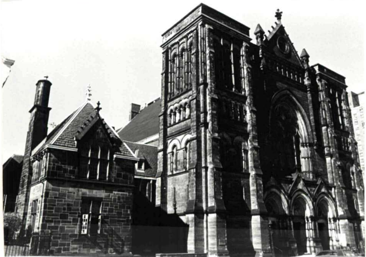
Emmanuel Baptist Church, 279-291 Lafayette Avenue. Francis H. Kimball, architect, 1866-1887.
