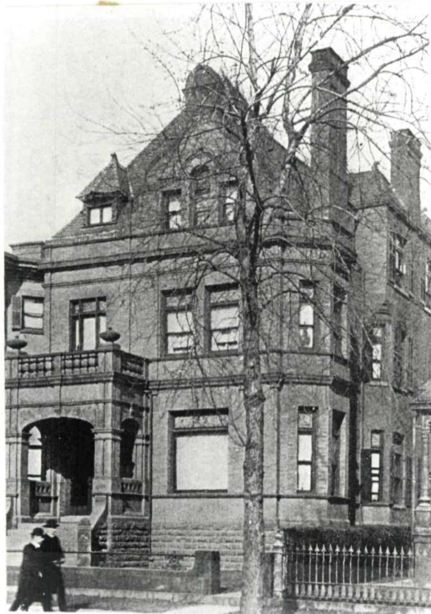
Chas. A. Schieren Residence, 405 Clinton Avenue. William Tubby, architect, 1889 (from: Kings Views of Brooklyn , 1904, p. 45).
