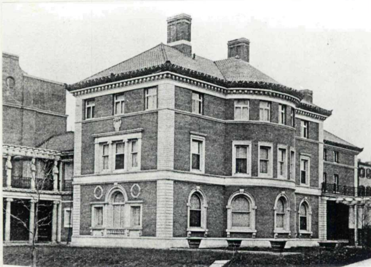
Frederick B. Pratt Residence, 229 Clinton Avenue. Babb, Cook & Willard, architects, 1895-97 (from: Kings Views of Brooklyn , 1904, p. 42).
