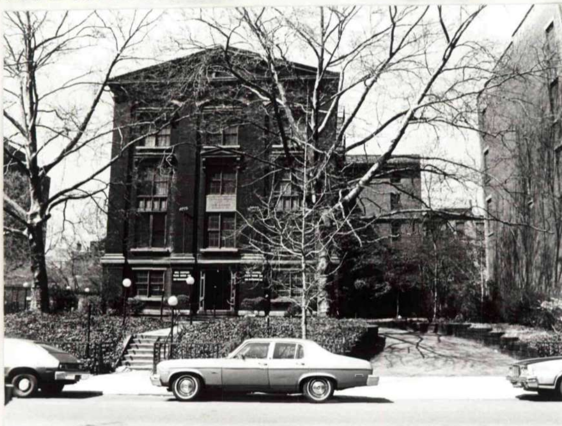
Graham Home for Old Ladies, 320 Washington Avenue. J.G. Glover, architect, 1851.
