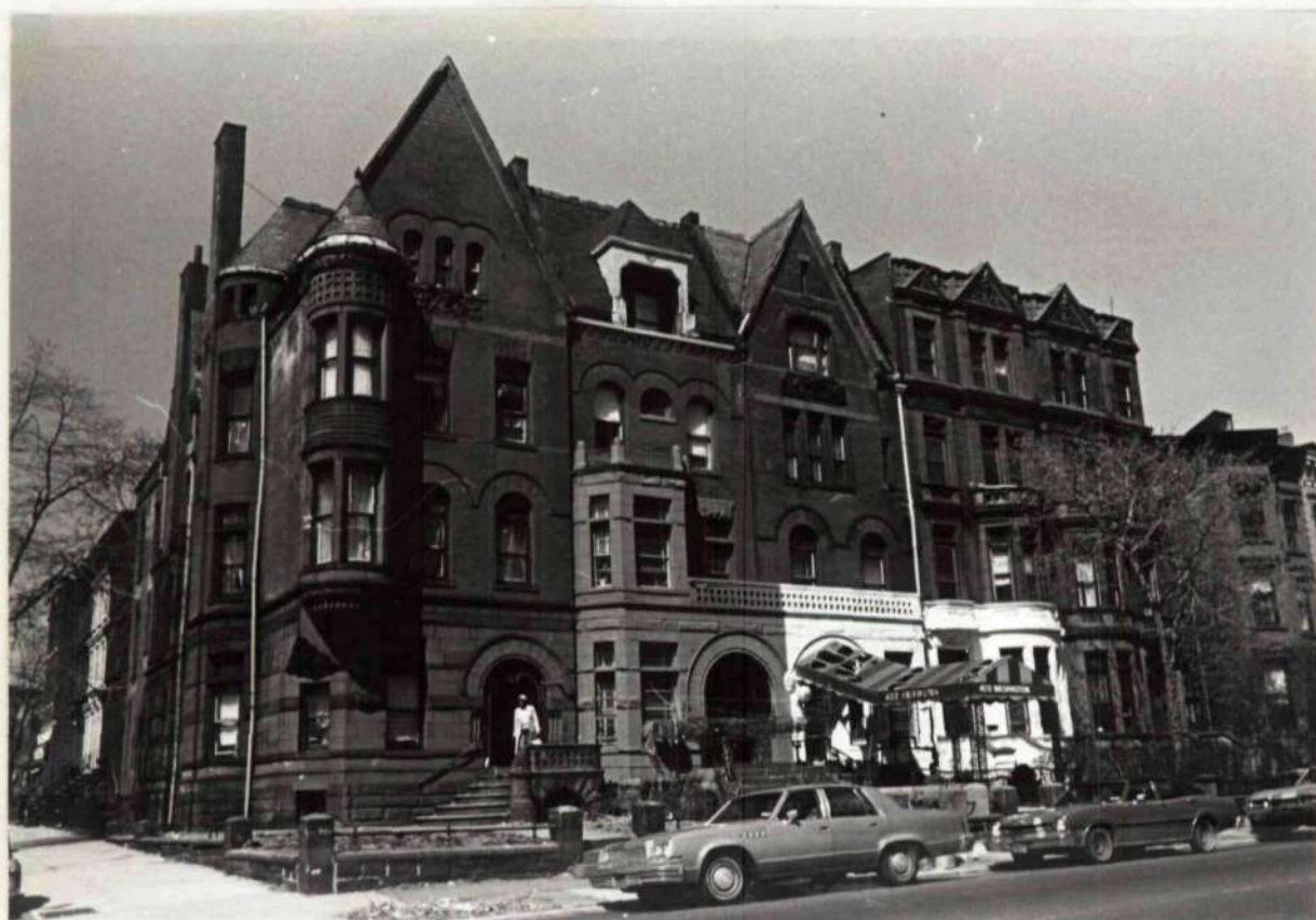
396-404 Washington Avenue. Adam E. Fisher, architect, 1887 and Mercein Thomas, architect, 1885. (photo reads from right to left)
