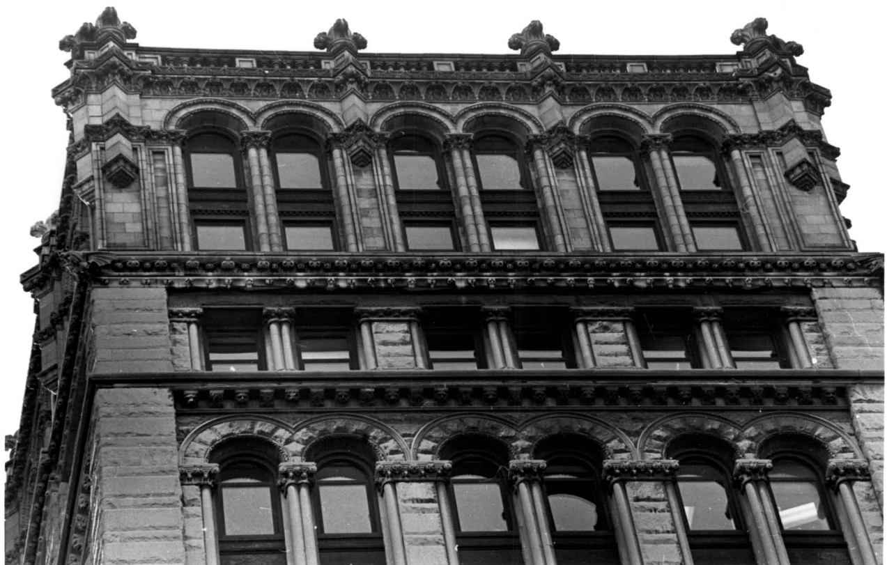
Details of the 1903-05 addition on Spruce Street Photos: Carl Forster
