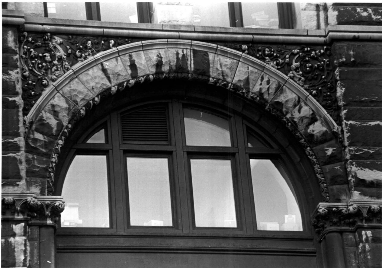
Top: Detail of a tenth-eleventh-story arcade, Park Row facade
