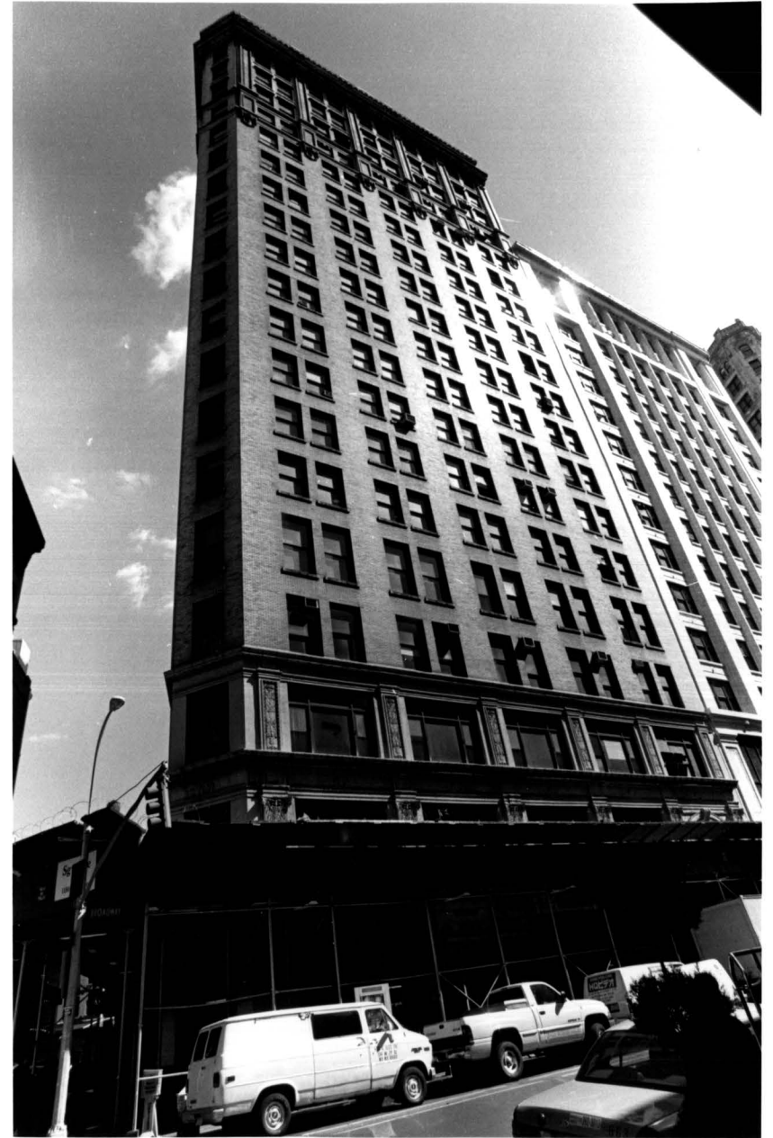
“The Victoria Building,” 228-232 Fifth Avenue, aka 2-4 West 27 th Street and 1148-1156 Broadway (Broadway facade) Photo: Carl Forster, 2001
