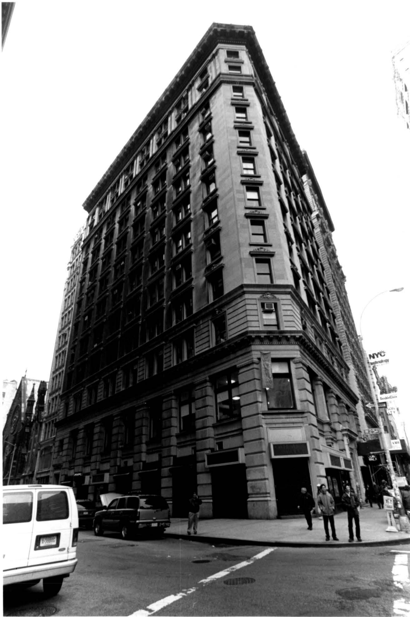
“The Townsend Building,” 1121-1127 Broadway, aka 9 West 25 th Street. Photo: Carl Forster, 2001
