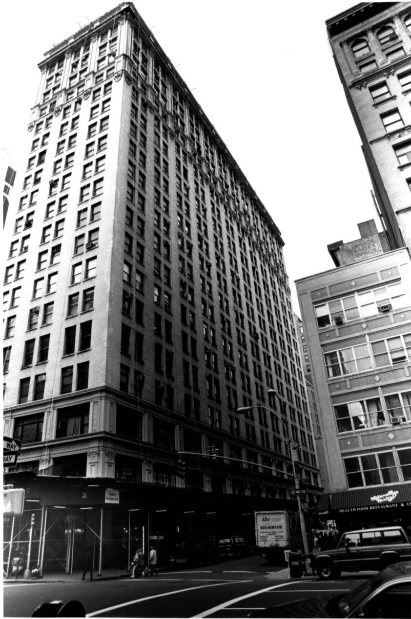
“The Victoria Building,” 228-232 Fifth Avenue, aka 2-4 West 27 th Street and 1148-1156 Broadway (Fifth Avenue and West 27 th Street facades) Photo: Carl Forster, 2001
