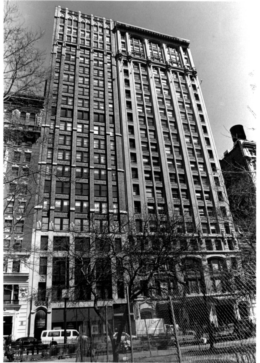
"The Goddard Building," 11-13 East 26 th Street, aka 6-8 East 27 th Street, and "The Madison Square Building," 15-19 East 26 th Street, aka 10-14 East 27 th Street. Photo: Carl Forster, 2001
