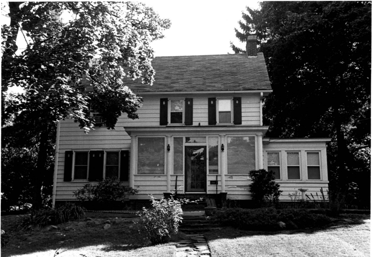
41-45 20 th Street. Built in the mid-nineteenth century with later alterations. Photo: Carl Forster, 2004.
