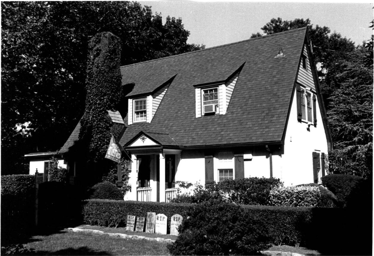
35 – 240 th Street (aka 41-10 – 41-14 20 th Street). Built c.1928. Photo: Carl Forster, 2004.
