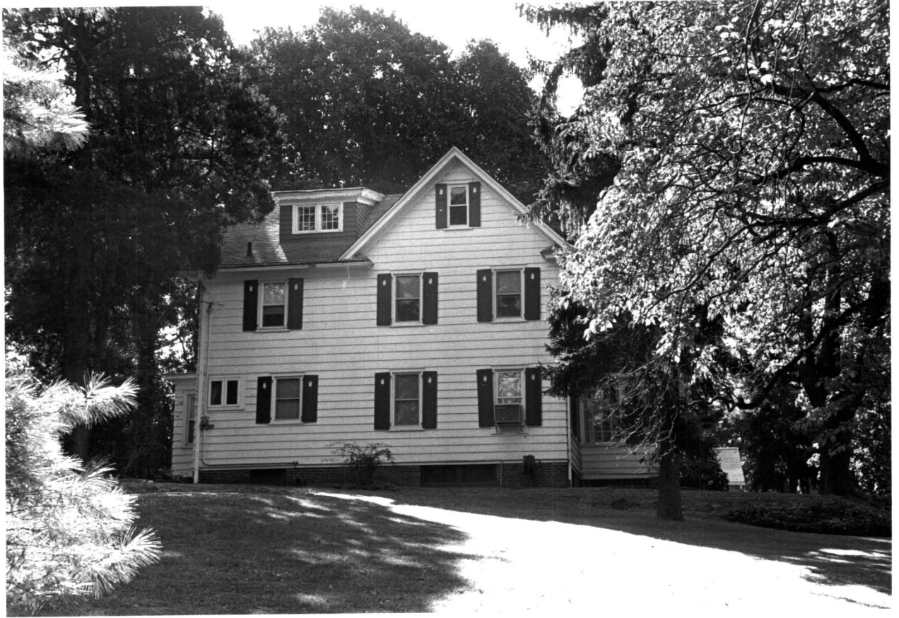
41-45 20 th Street. Depew Avenue façade. Photo: Carl Forster, 2004.
