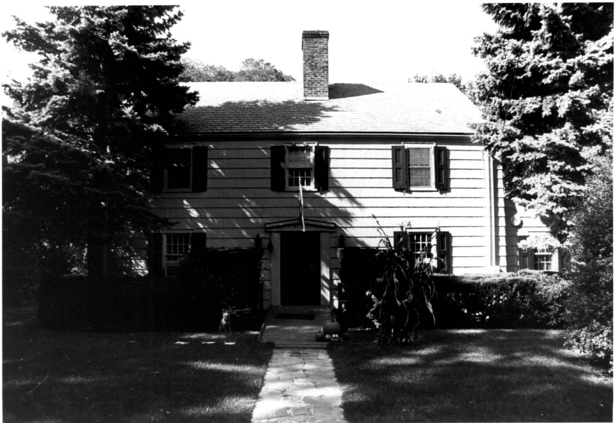
41-18 240 th Street (aka 33 – 240 th Street). Built c.1928. Photo: Carl Forster, 2004.
