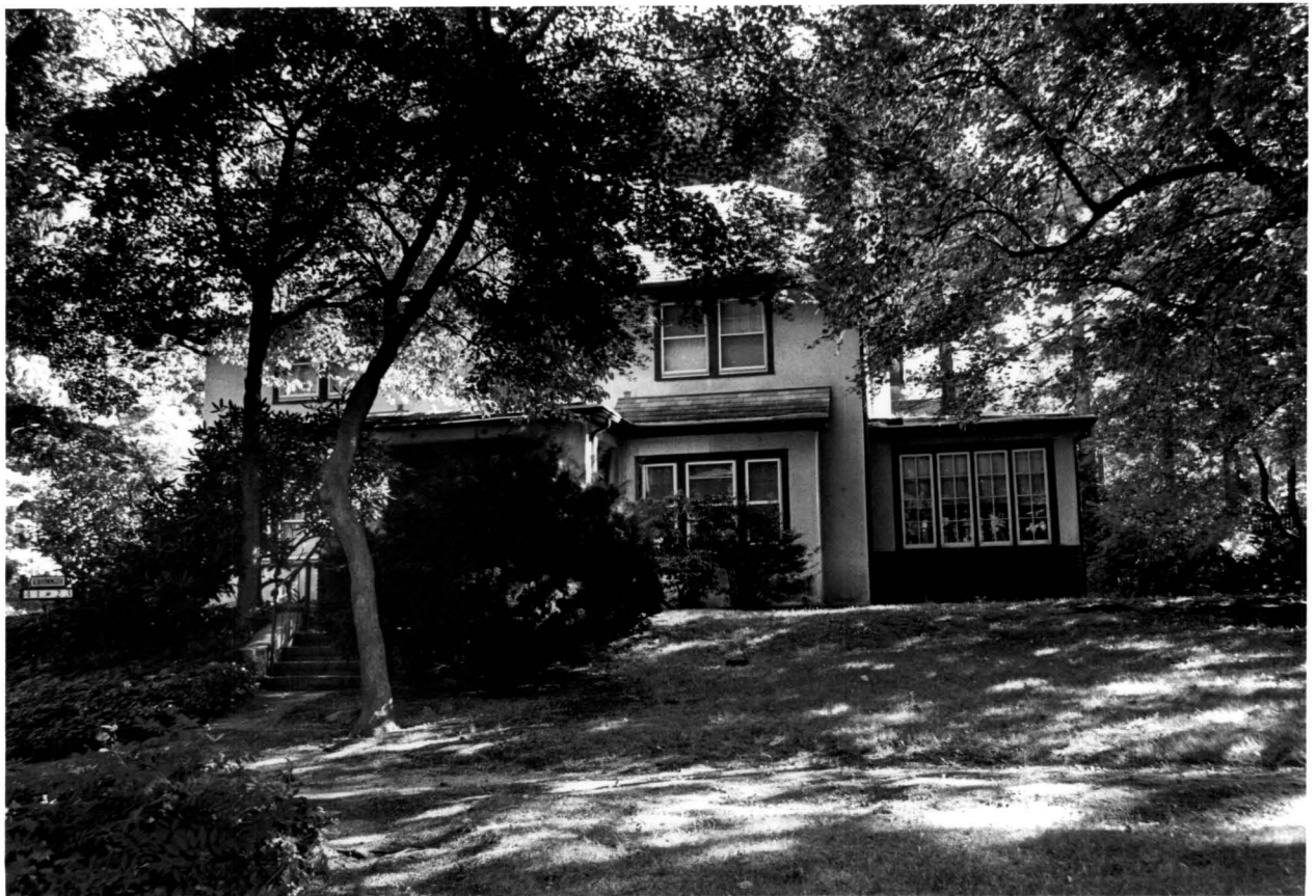
240-01 42 nd Avenue (aka 41-23 240 th Street and 22 – 240 th Street). Built 1921. Photo: Carl Forster, 2004.
