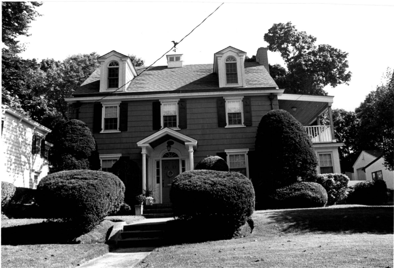
42-09 240 th Street (aka 42-11 240 th Street and 16 – 240 th Street). main façade . Built 1926. Samuel Lindbloom, architect. Photo: Carl Forster, 2004.
