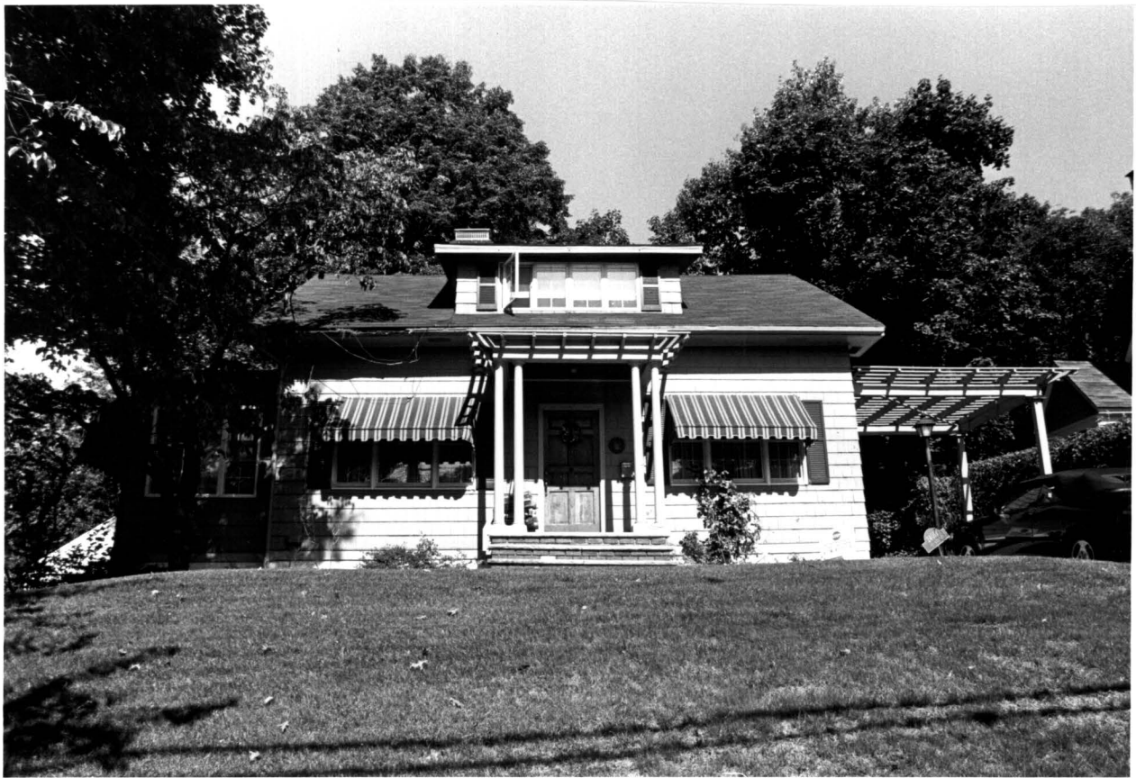
240-11 43 rd Avenue. Built 1926-27. Aubrey B. Grantham, architect. Photo: Carl Forster, 2004.
