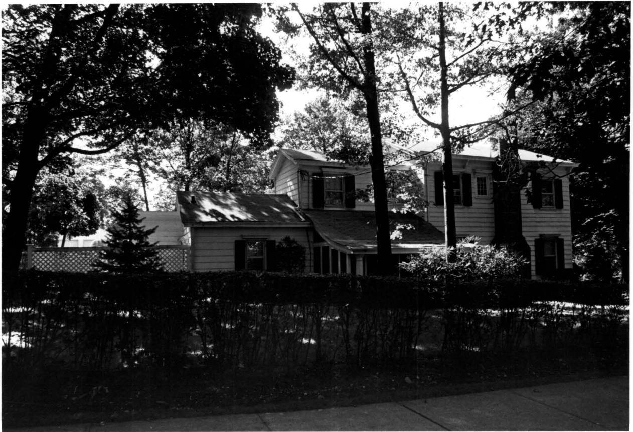
240-02 42 nd Avenue (aka 42-01 240 th Street). Built c.1850, moved to this location and altered in 1927. Samuel Lindbloom, architect (1927). Photo: Carl Forster, 2004.
