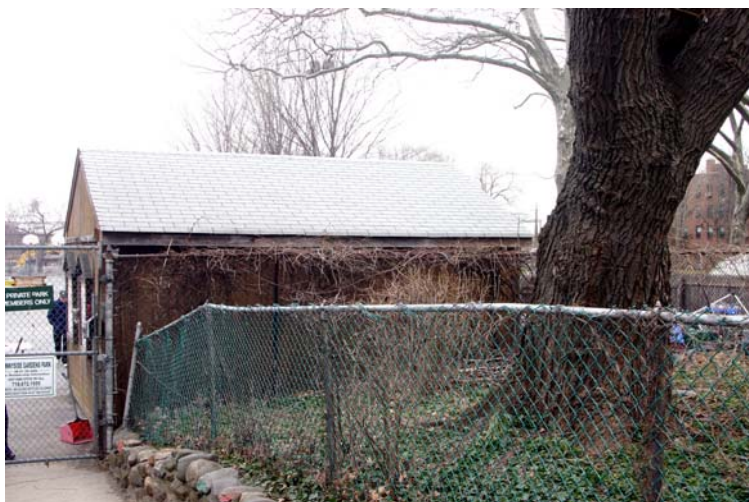
West and south facades of office building
