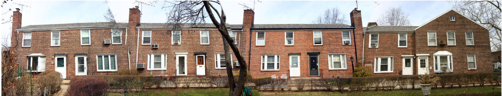
39-88 44 th St 39-86 44 th St 39-84 44 th St 39-82 44 th St 39-80 44 th St 39-78 44 th St 39-76 44 th St 39-74 44 th St
