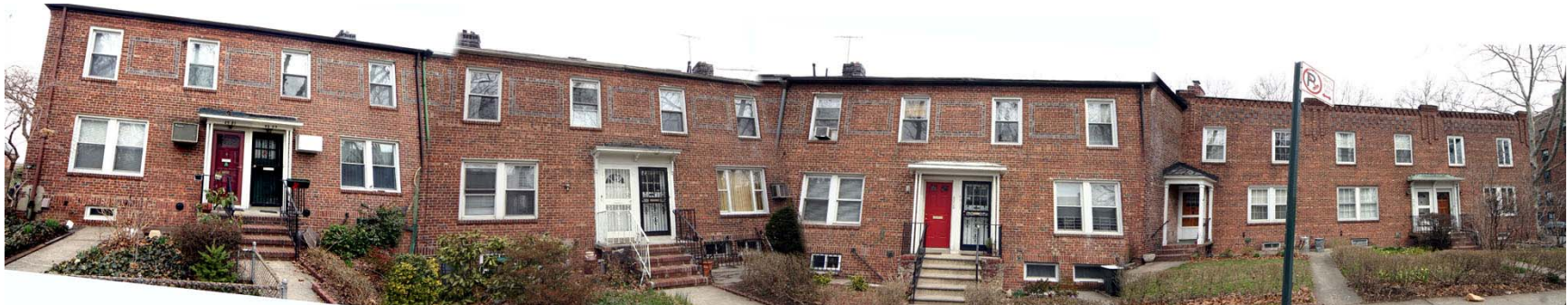
49-01 39 th Ave 49-03 39 th Ave 49-05 39 th Ave 49-07 39 th Ave 49-09 39 th Ave 49-11 39 th Ave 49-13 39 th Ave 49-15 39 th Ave 49-17 39 th Ave
