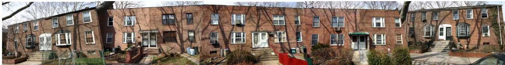
40-30 44 th St 40-28 44 th St 40-26 44 th St 40-22 44 th St 40-20 44 th St 40-18 44 th St 40-16 44 th St 40-14 44 th St 40-12 44 th St 40-10 44 th St
