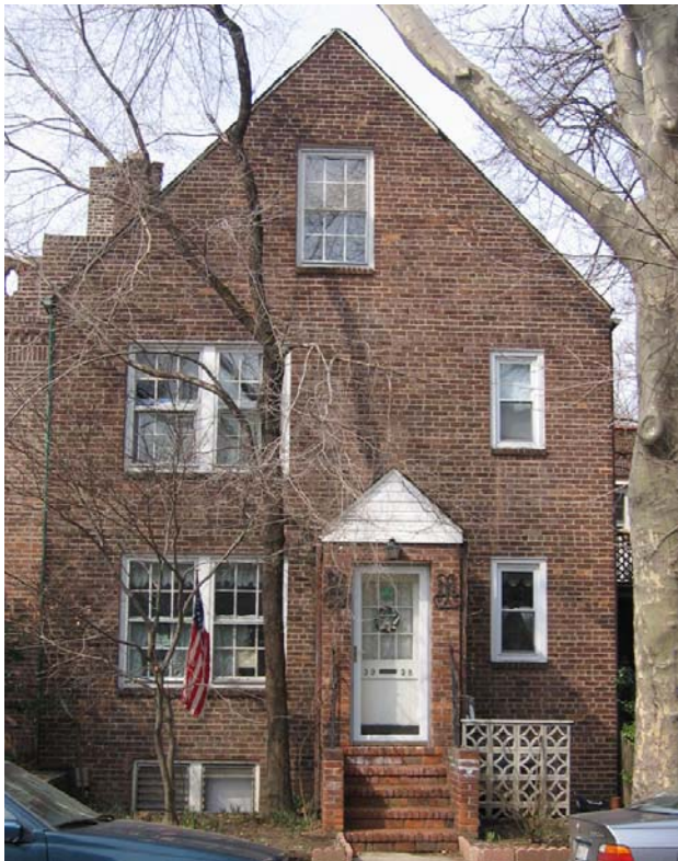
39-58 47 th Street – non-historic porch infill
