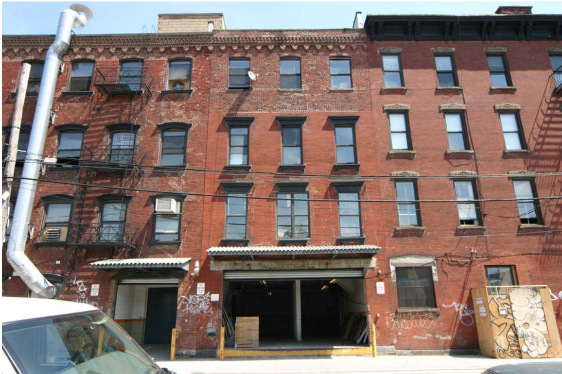
98 West Street (at center of view)
