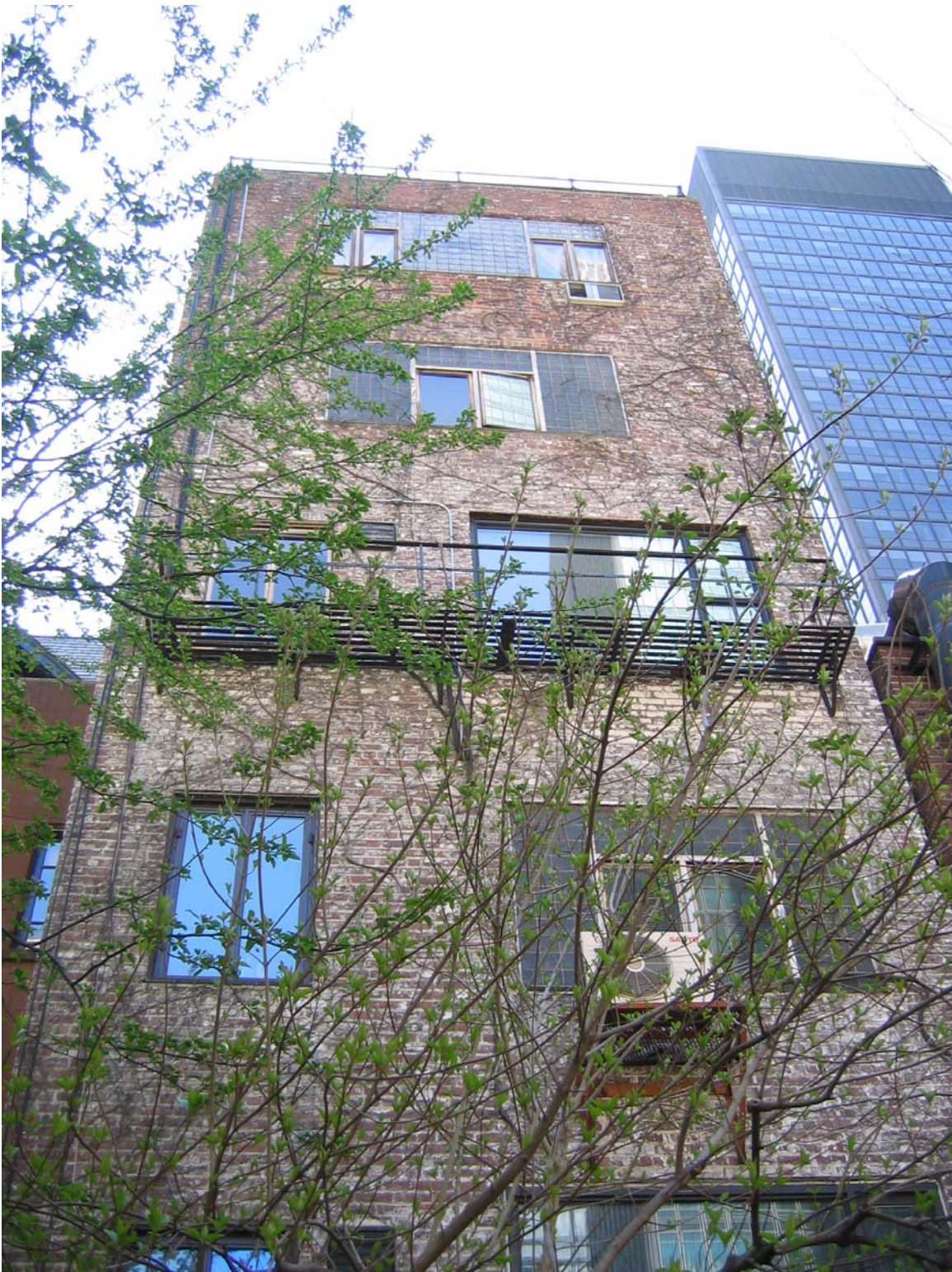
Morris B. Sanders Studio & Apartment Rear facade, view from Amster Yard Photo by Matthew A. Postal
