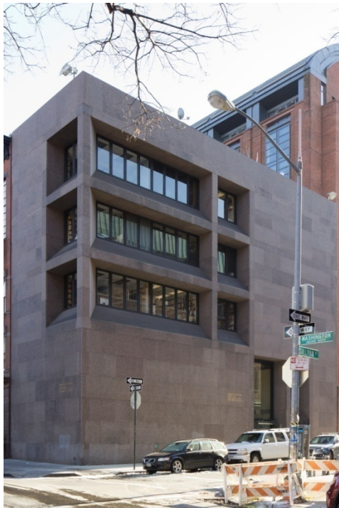
Hagop Kevorkian Center for Near Eastern Studies , 50 Washington Square South Built in 1969-72 and designed by Philip Johnson and Richard Foster
