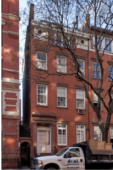
132 West 4 th Street Built c. 1839, renovated in 1917 during alterations designed by Josephine Wright Chapman
