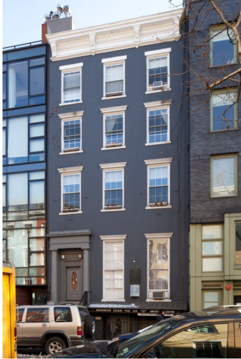
179 Sullivan Street Built c. 1834 as part of the Varick Place residential terrace, raised to four full stories in 1879
