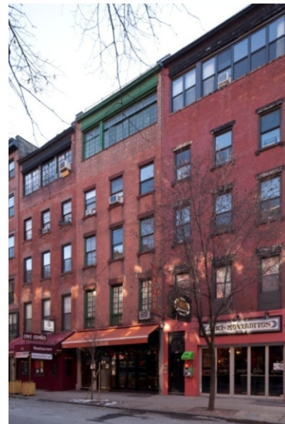
172 to 176 Bleeker Street The row was updated in the 1920s with studio windows and other alterations Photo: Christopher D. Brazee (December 12, 2013)
