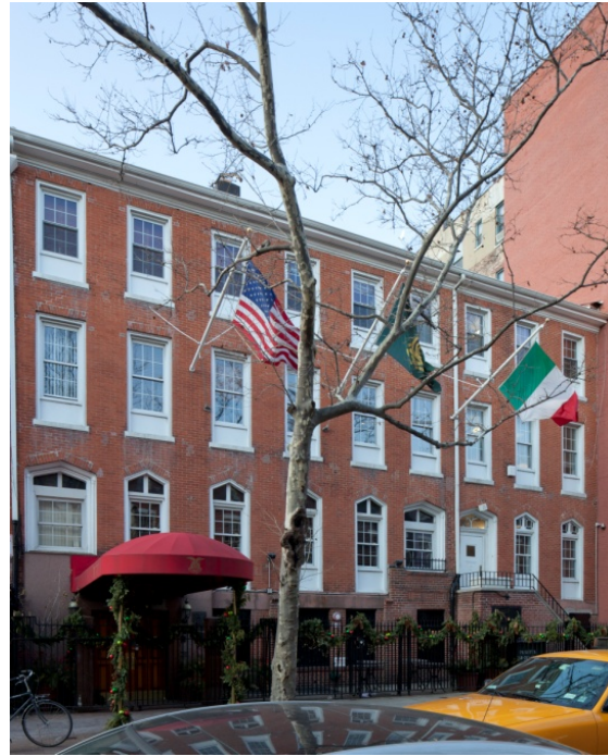
73 to 77 MacDougal Street Photo: Christopher D. Brazee (December 12, 2013)
