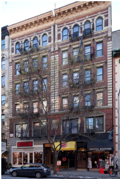
192 and 194 Bleecker Street Built in 1901 and designed by John P. Cleary
