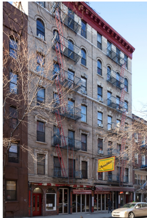
103 and 105 MacDougal Street Built in 1901-02 and designed by Michael Berstein
