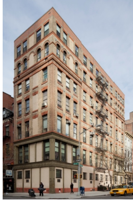
520 LaGuardia Place Built in 1890 and designed by Cleverdon & Putzel
