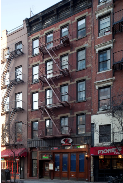
167 Bleecker Street Built 1886-87 and designed by John B. Snook
