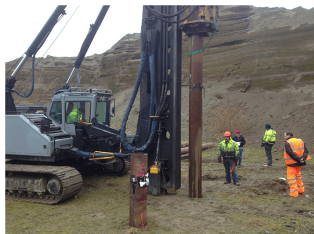
Fig. 1. Driving of the FBG test pile
