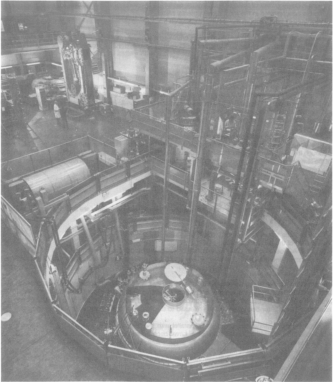
"TOSKA" Facility at Kernforschungszentrum Karlsruhe (KfK)
