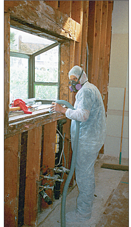
Although the level of health risk presented by mold may not be fully understood, remediation workers involved in more serious cases may be required to wear personal protective gear.
