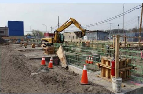
May 2016 – Installation of formwork, rebar and foundation at the EMU (Electric Multiple Unit) Annex.
