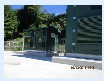
New 2.3MVA Rectifier, and 112.5 KVA Auxiliary Cast-Coil Transformer
