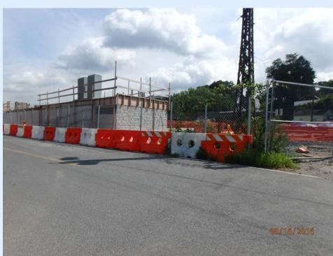
Elevated vault foundation for new A-25 Tarrytown substation
