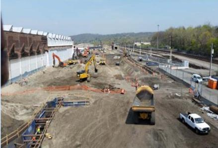
May 2016 - Consist Shop facility concrete floor slabs, excavations and installation of electrical duct banks, water and storm drains utilities.
