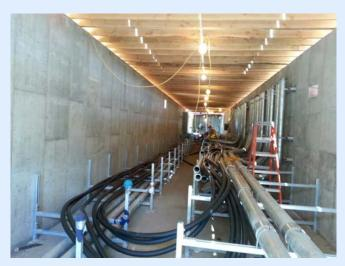
Elevated vault foundation for new A-33 Harmon Substation
