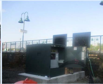
Pad-Mounted Electric Switch (PME ) for new 13.2 KV utility service connection
