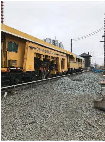
Realignment/Resurfacing of Track 10 by LIRR Forces
