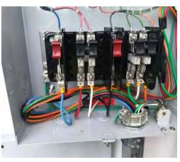
Meter pan wire harness installation at Riverdale and Tarrytown Substations.
