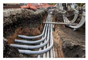
Hastings - Sectionalizing switch & traction power system conduits.
