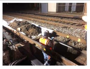
*Night Work:* Phase IB – Hastings-on-Hudson North of CP19 Greystone - Crossing for track 2 Impedance bond conduits installation for traction power negative returns.
