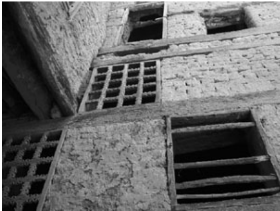
Figure 7: Screening wooden elements
