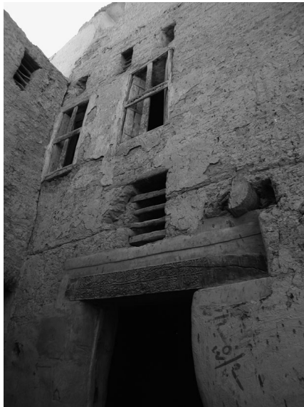
Figure 4: The house surveyed in Al Qasr
