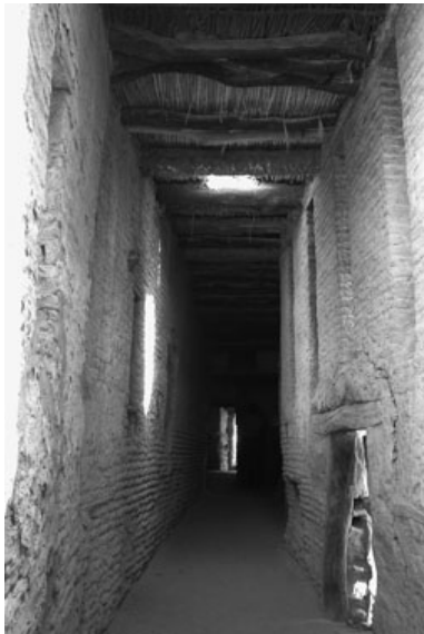
Figure 2: A covered street in Al Qasr
