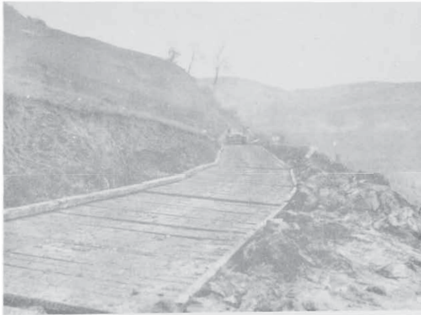
PLANK ROAD BUILT BY 109TH NEAR LOIANO
