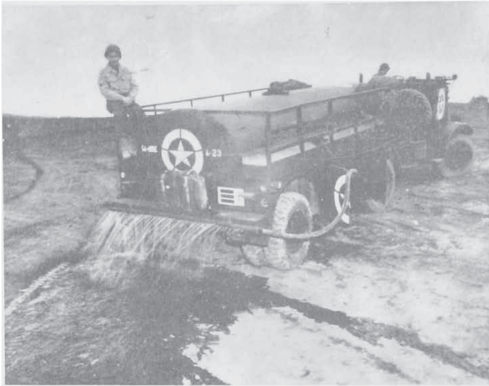
405TH TANKER SPRINKLING AN AIRFIELD
