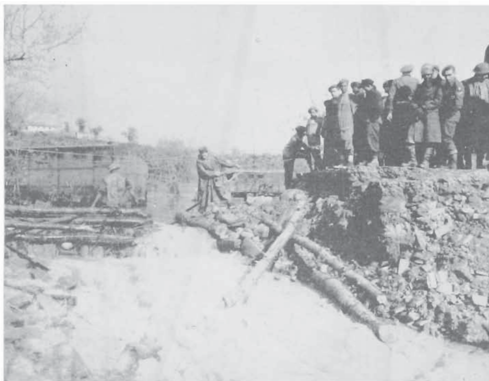
INDIAN ENGINEERS PREPARING BRIDGE SITE NEAR BORGIO SAN LORENZO
