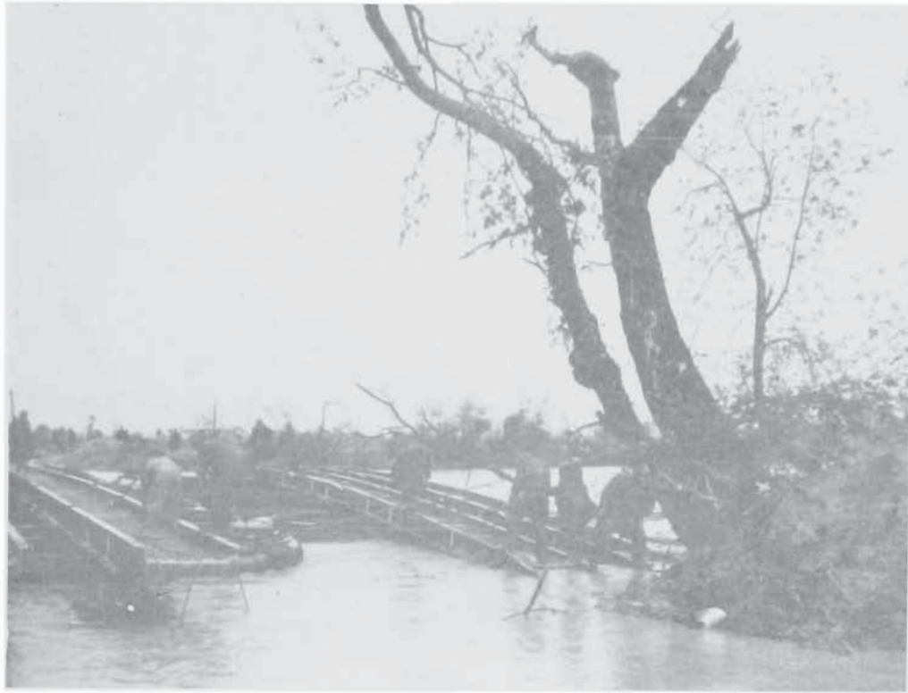
16TH ENGINEERS TRY TO SAVE TREADWAY
