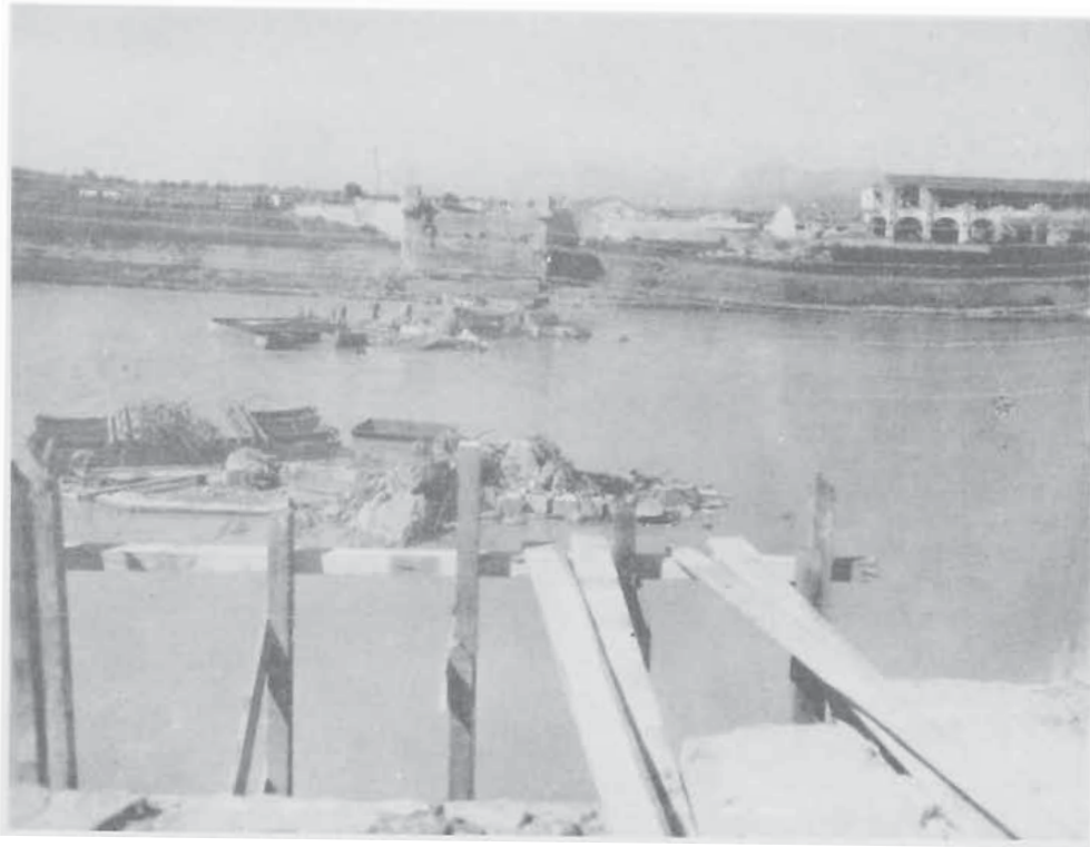
DEMOLISHED BRIDGE AT PISA
