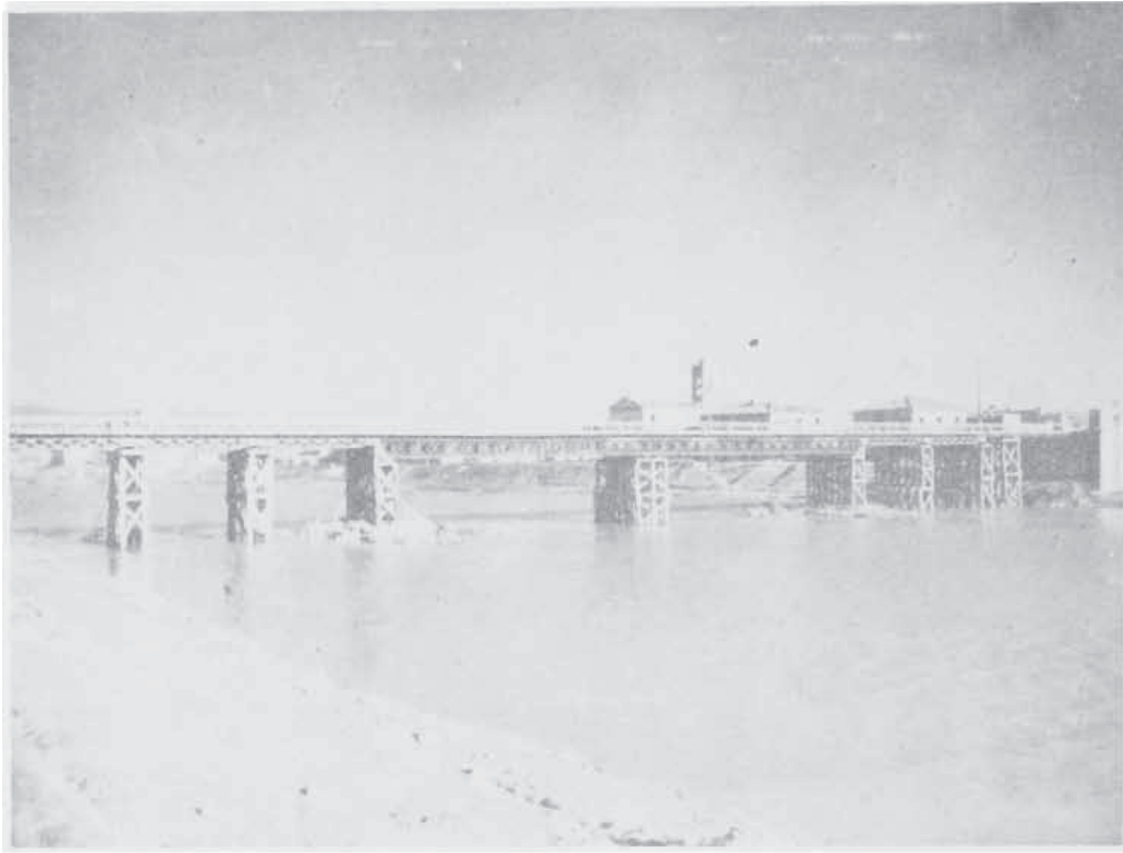
THE FINISHED BRIDGE
