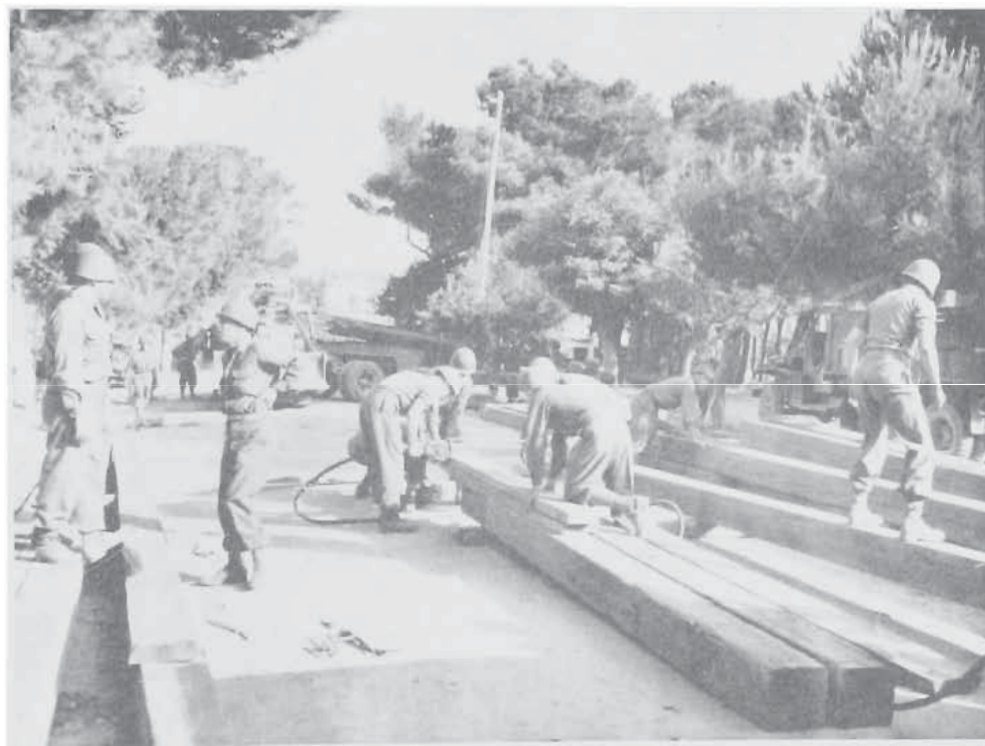
310TH ENGINEERS CUTTING BRIDGE TIMBERS IN LEGHORN AREA
