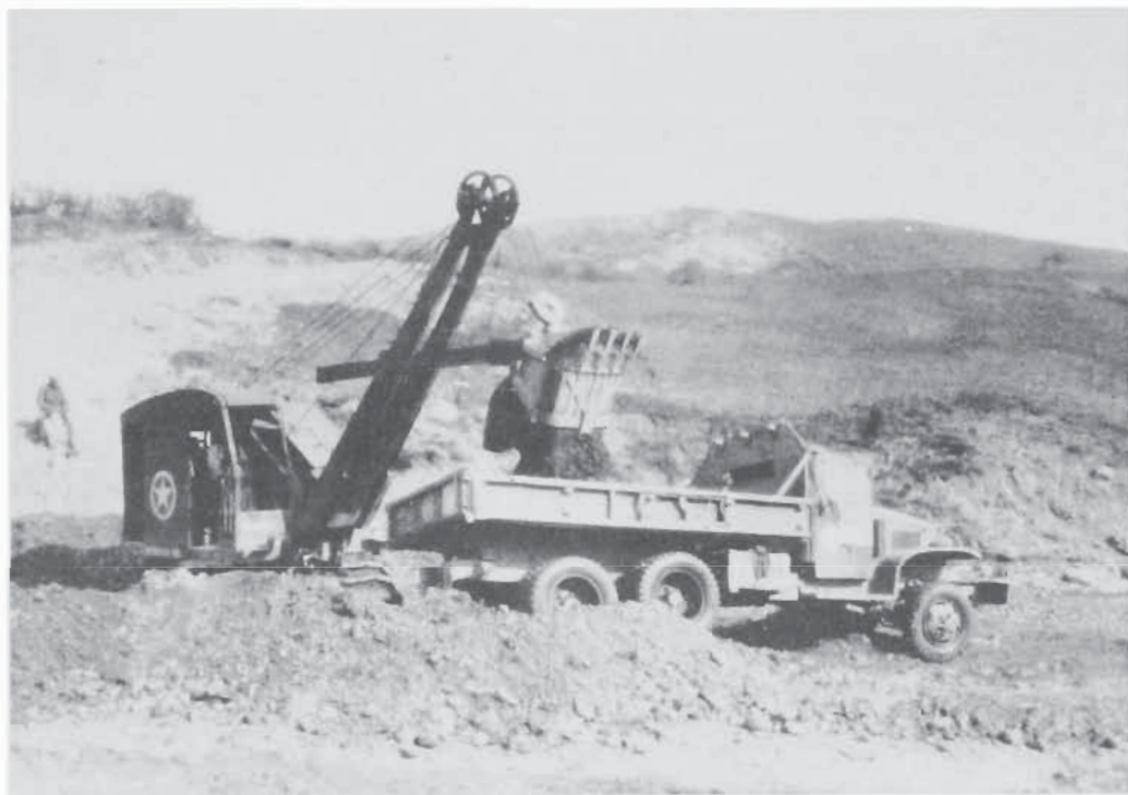
LOADING UP DUMP TRUCK SOUTH OF BOLOGNA
