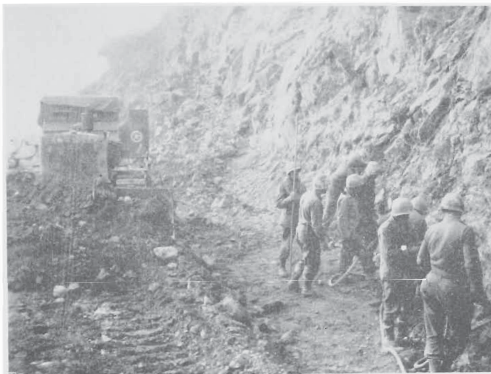
310TH PREPARING BLAST HOLES IN QUARRY NEAR BACCANELLO
