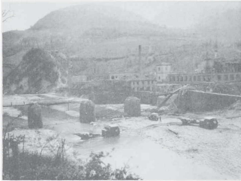
RENO RIVER FORD BUILT BY SOUTH AFRICAN ENGINEERS
