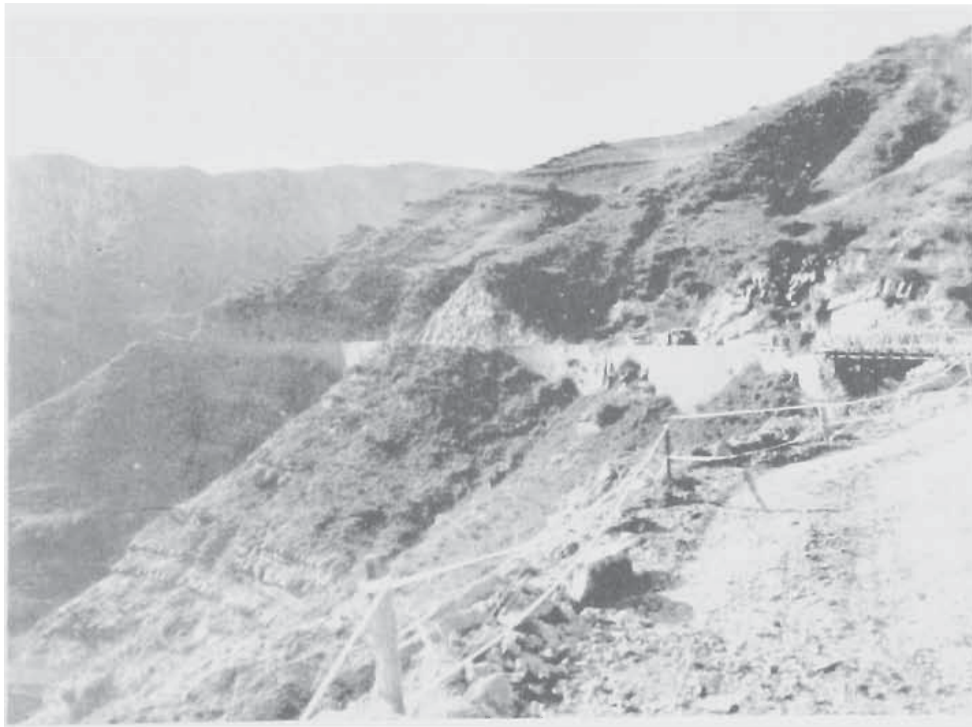
BYPASS BUILT BY THE 1ST BRITISH DIVISION ENGINEERS
