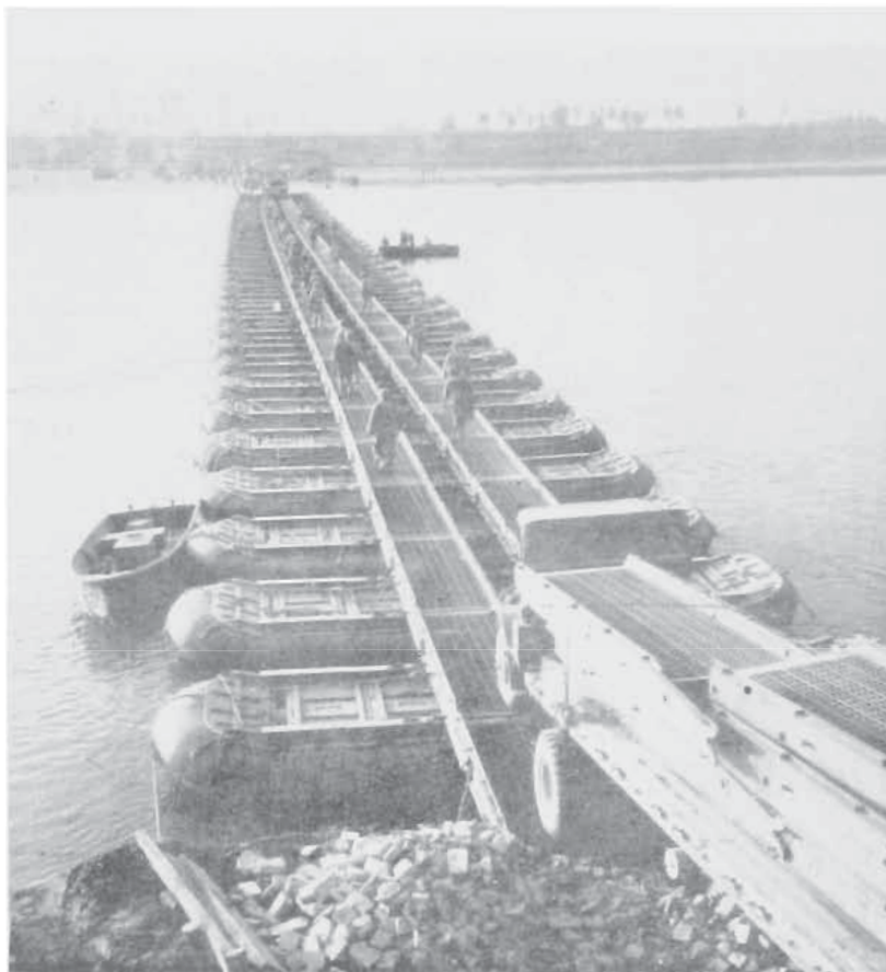
THE 402ND BRIDGE ACROSS THE PO NEAR OSTIGLIA
