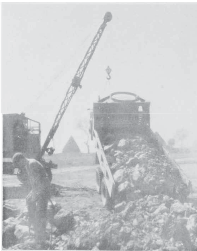
CRANE PLUS GMC EQUALS DUMP TRUCK FOR THE 16TH ENGINEERS WORKING ON NERO'S PIKE NEAR ANZIO
