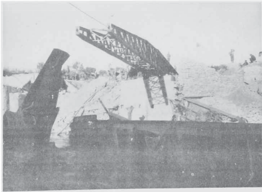
RAILROAD BRIDGE NEAR PISTOIA UNDER CONSTRUCTION BY 182ND ENGINEERS
