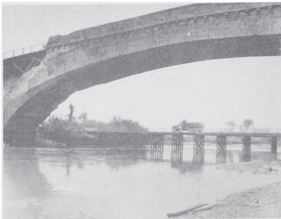
THE 337TH'S BRIDGE ACROSS THE SELE--ORIGINAL BRIDGE IN FOREGROUND
