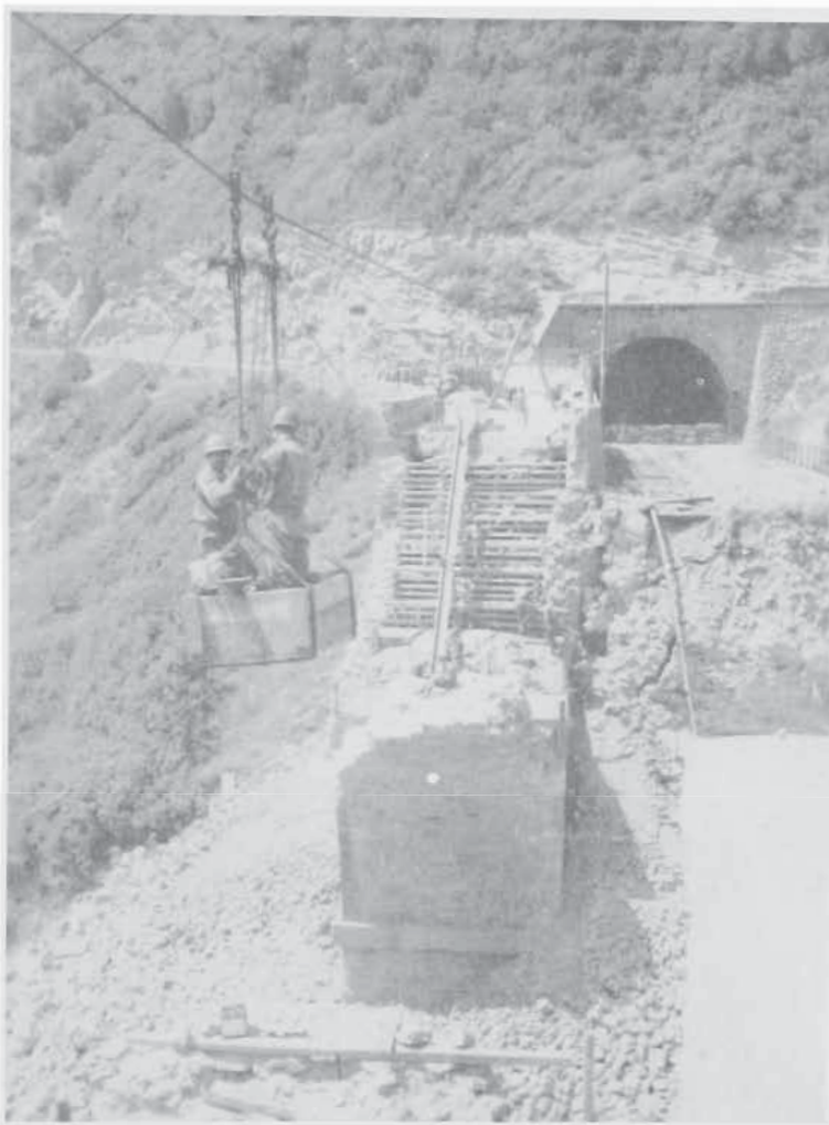
CABLE CAR USED BY 175TH IN CONSTRUCTION OF BRIDGE NEAR LEGHORN
