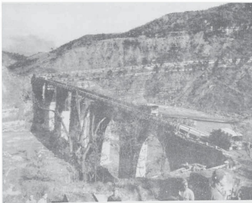
BAILEY BUILT BY 56TH FIELD COMPANY NEAR SAN ANDREA
