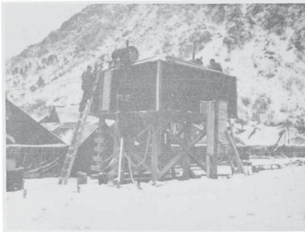
WINTERIZED WATER TOWER BUILT BY 405TH
