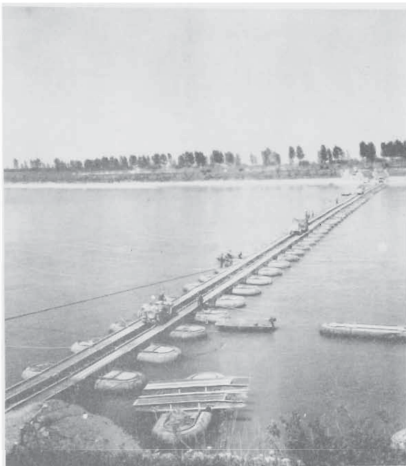
PO RIVER BRIDGE NEAR BREDE BUILT BY 401ST ENGINEERS
