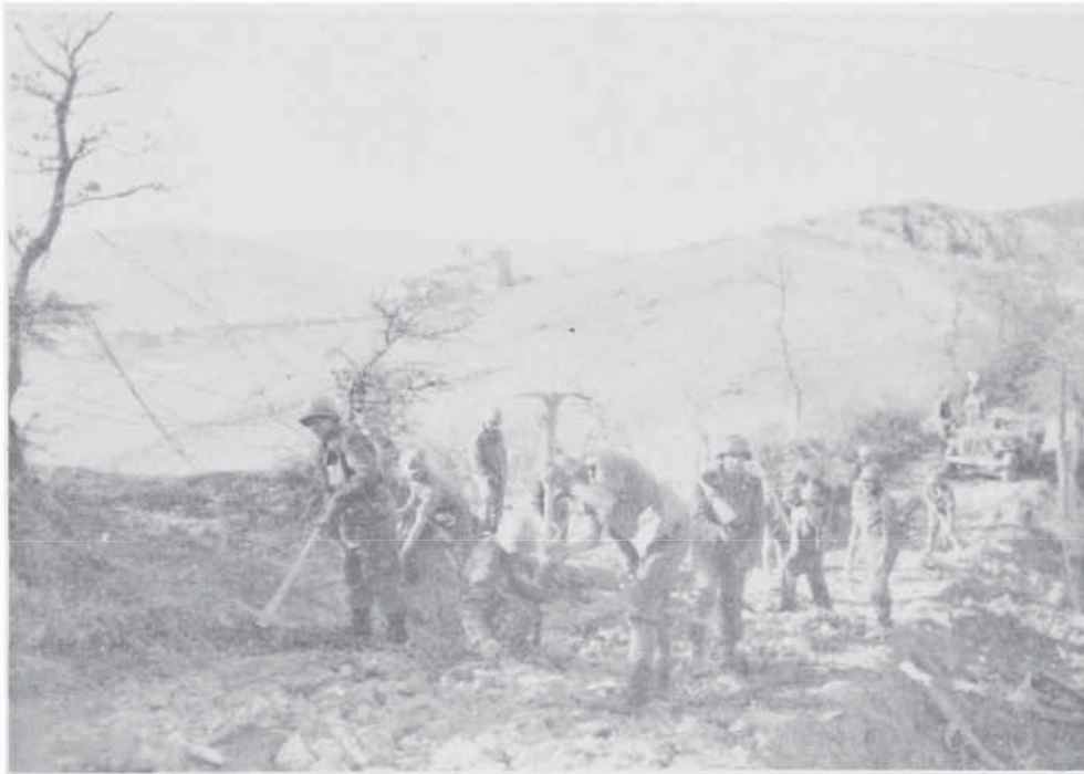
BRAZILIAN ENGINEERS BUILDING ROAD NEAR SILLA
