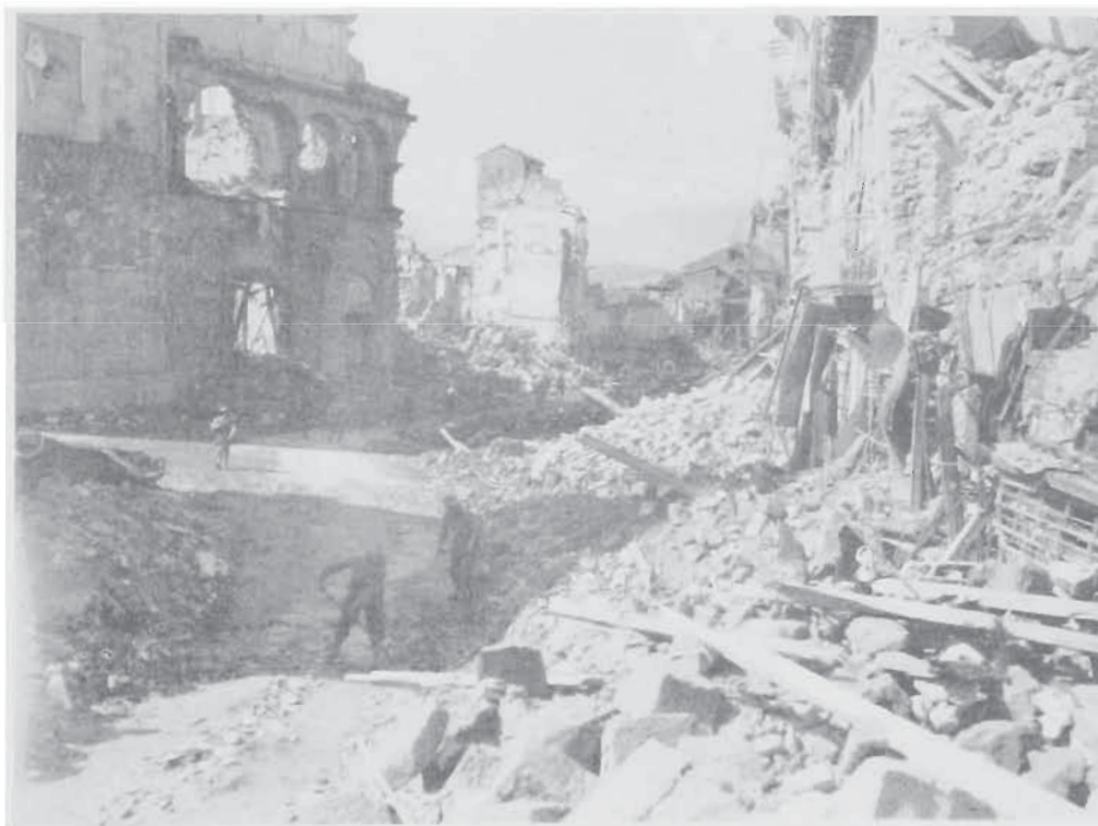
RUBBLE CLEARING OPERATIONS
