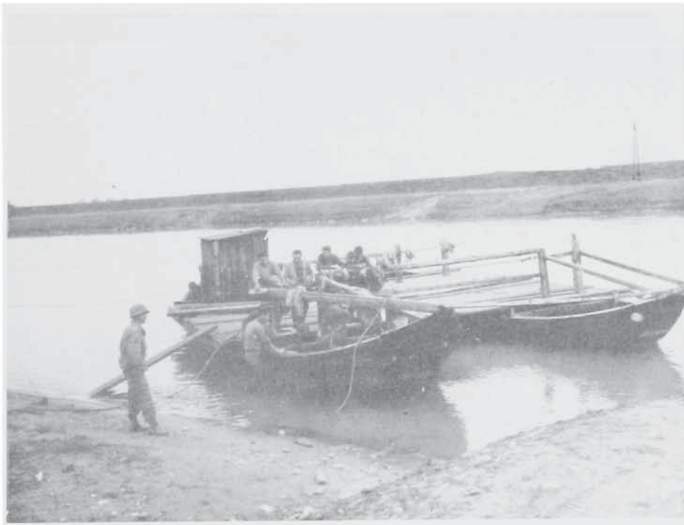
IMPROVISED CLASS 30 RAFT BUILT BY 39TH ON THE ADIGE RIVER
