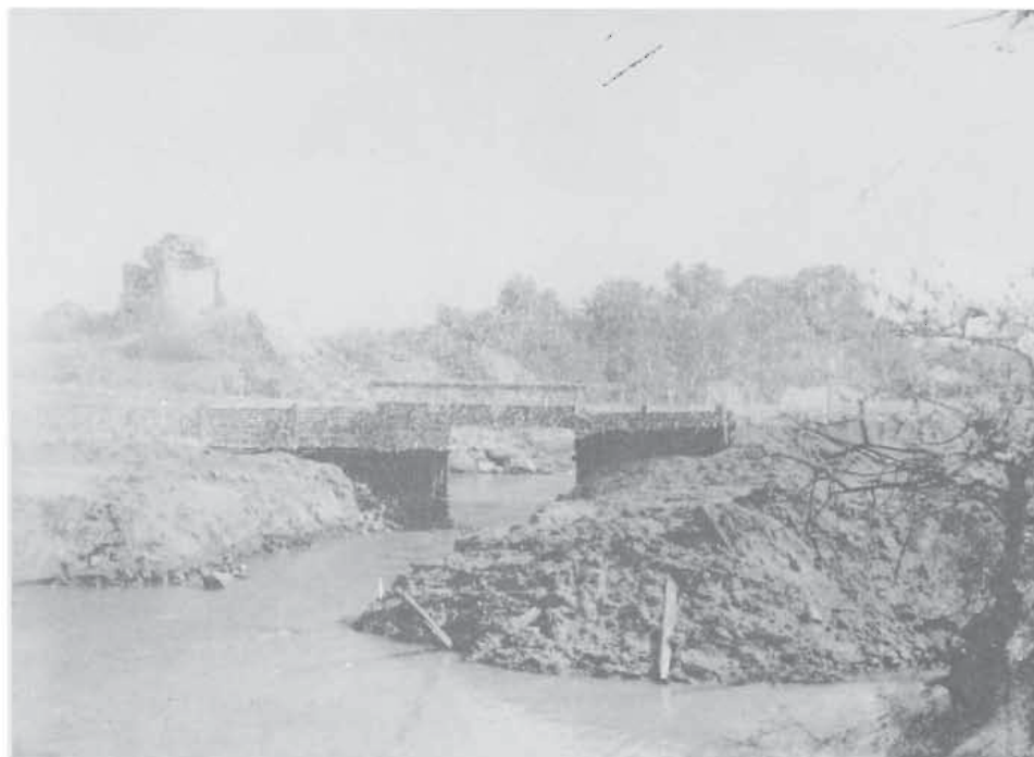
SMALL BRIDGE NEAR GROSSETTO CONSTRUCTED BY 337TH
