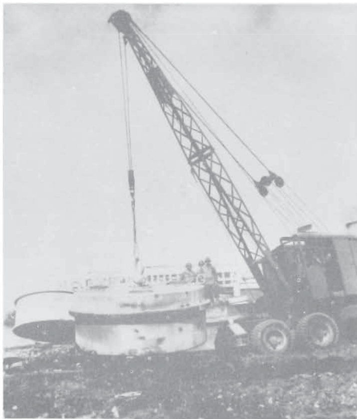
540TH ENGINEERS CLEARING NAPLES
