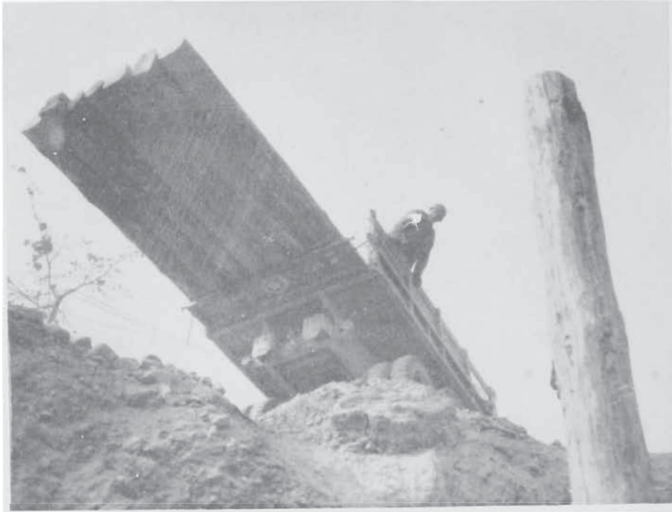
316TH BRINGS PILES FOR BRIDGE NEAR GOTHIC LINE
