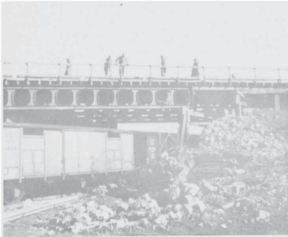
92ND ENGINEERS BUILDING OVERPASS NEAR CAPUA
