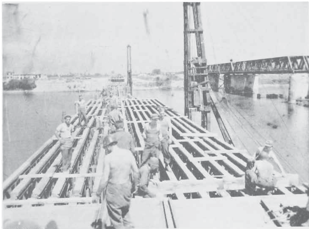
175TH BRIDGE ACROSS PO UNDER CONSTRUCTION
