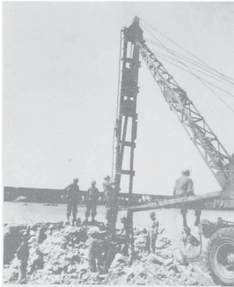
540th CONSTRUCTING PIER AT CIVITAVECCHIA
