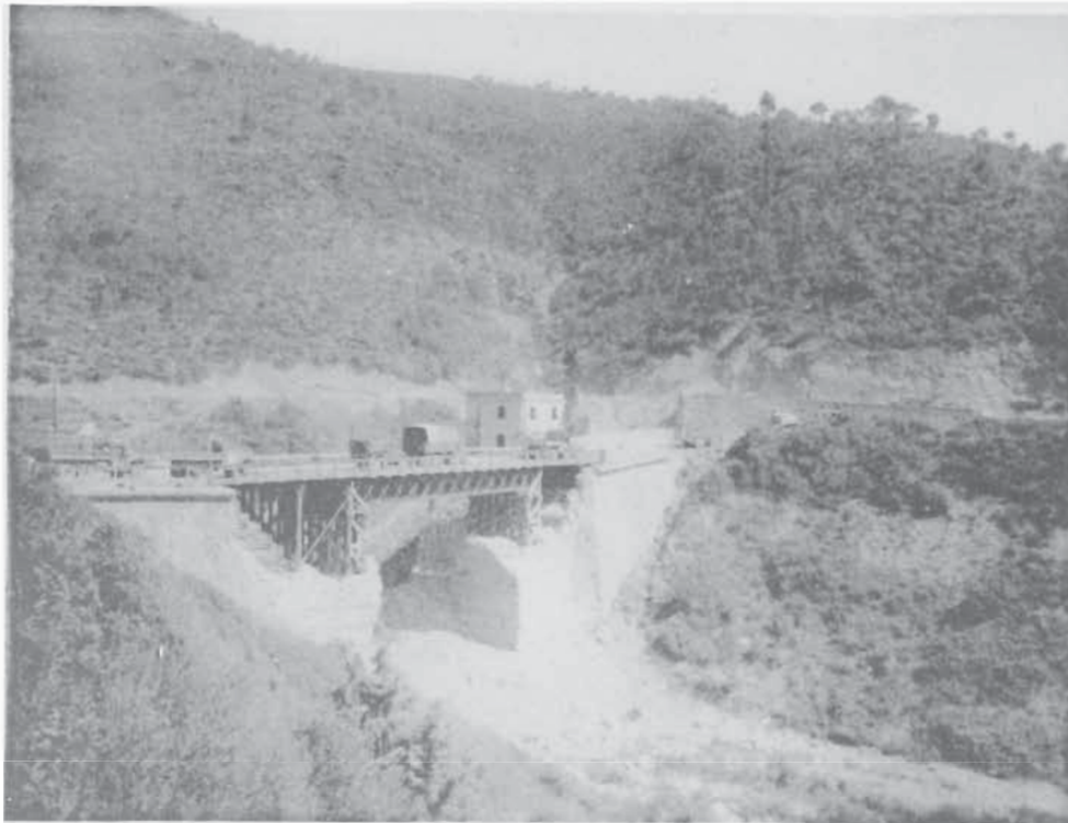
TIMBER TRESTLE BRIDGE WITH BAILEY GIRDERS BUILT BY 175TH ON ROUTE #1
