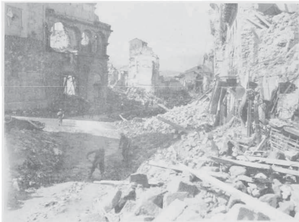
RUBBLE CLEARING OPERATIONS
