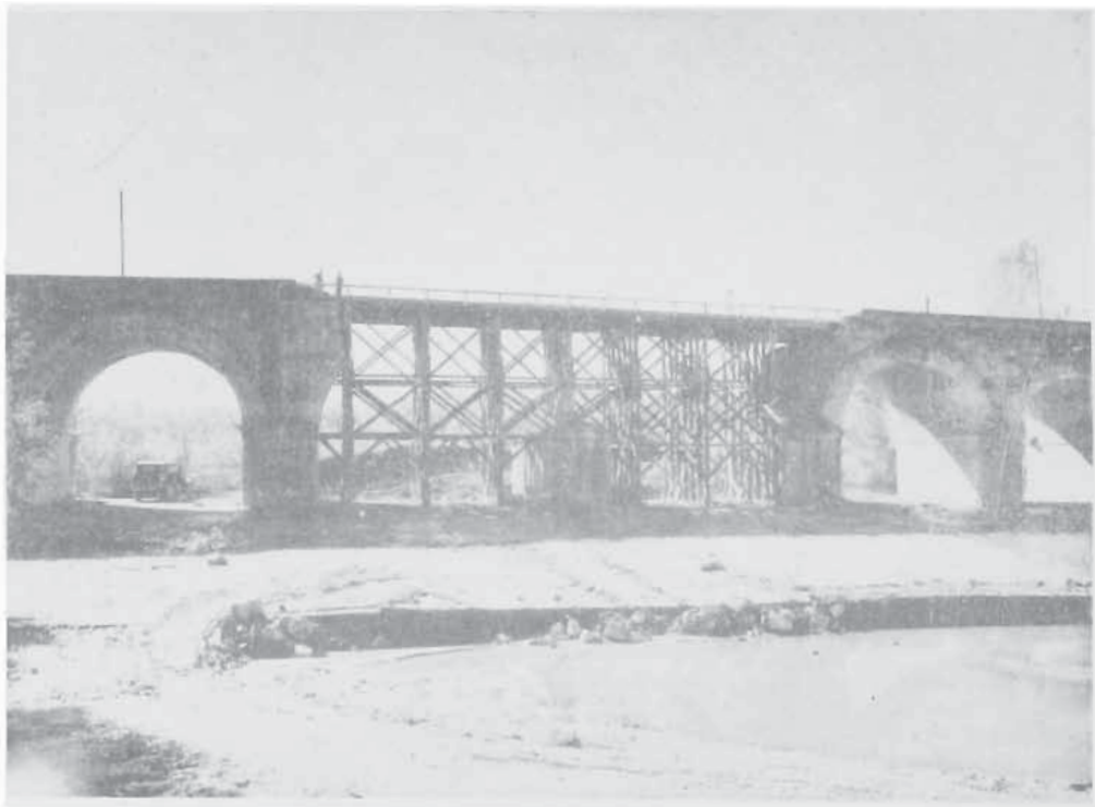
33 RD 'S BRIDGE AT GOTTOMINARDO
