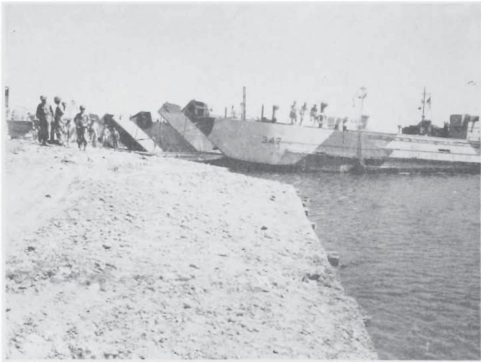
LCT HARDS BUILT BY 39TH AT PIOMBINO
