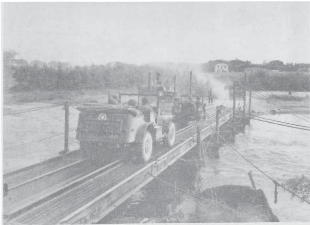
16TH'S FIXED TREADWAY BRIDGE OVER SELE RIVER
