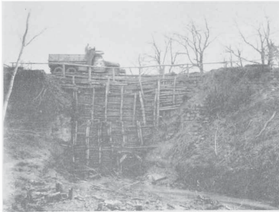
19TH ENGINEER CULVERT NEAR TEANO
