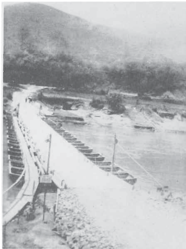
85TH ENGINEER HEAVY PONTON BRIDGE ACROSS GARIGLIANO
