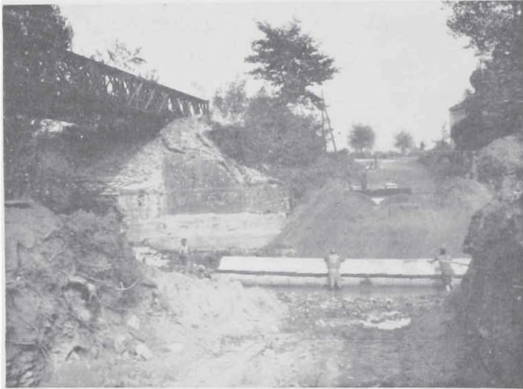
39TH PLACING CULVERT NEAR CAVALLINA
