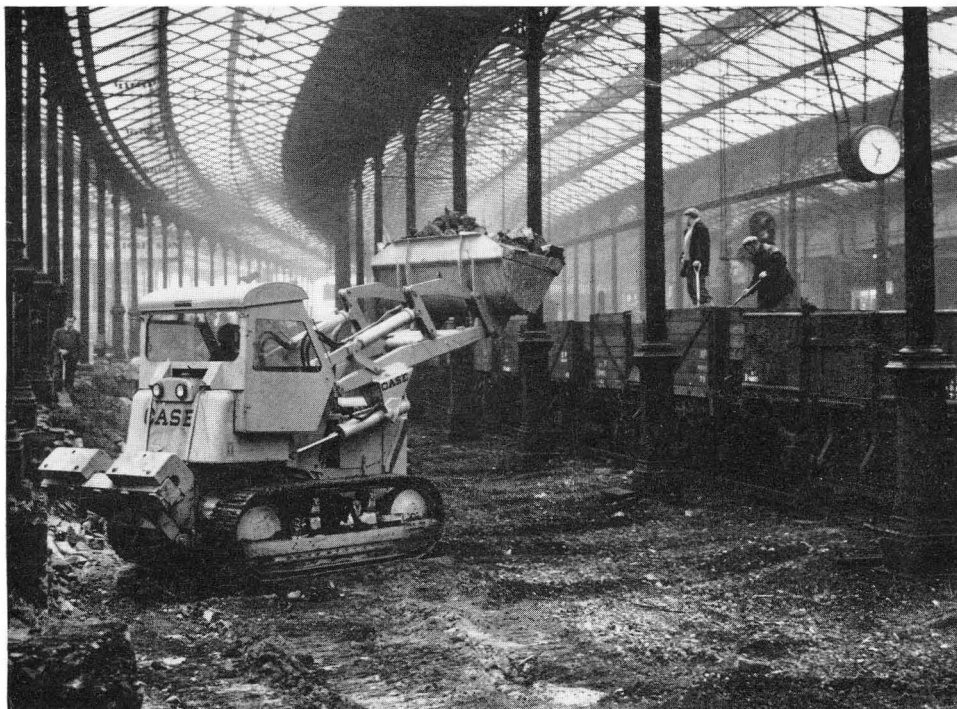
Work starts on new platform. February 1963
