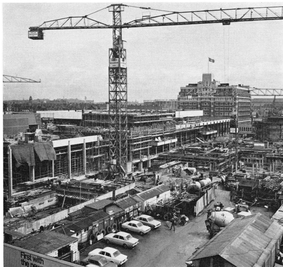
The frontage in the latter stages of construction
