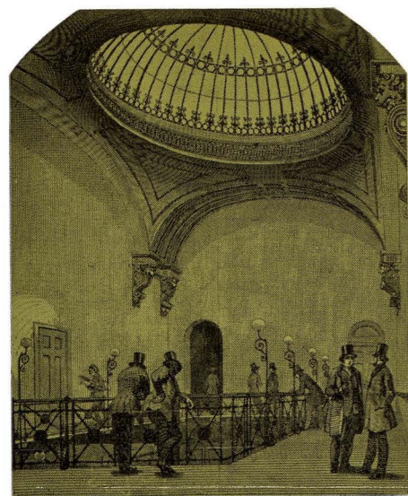
The gallery above the booking office at Euston. This ran parallel to the gallery which surrounded the Great Hall
