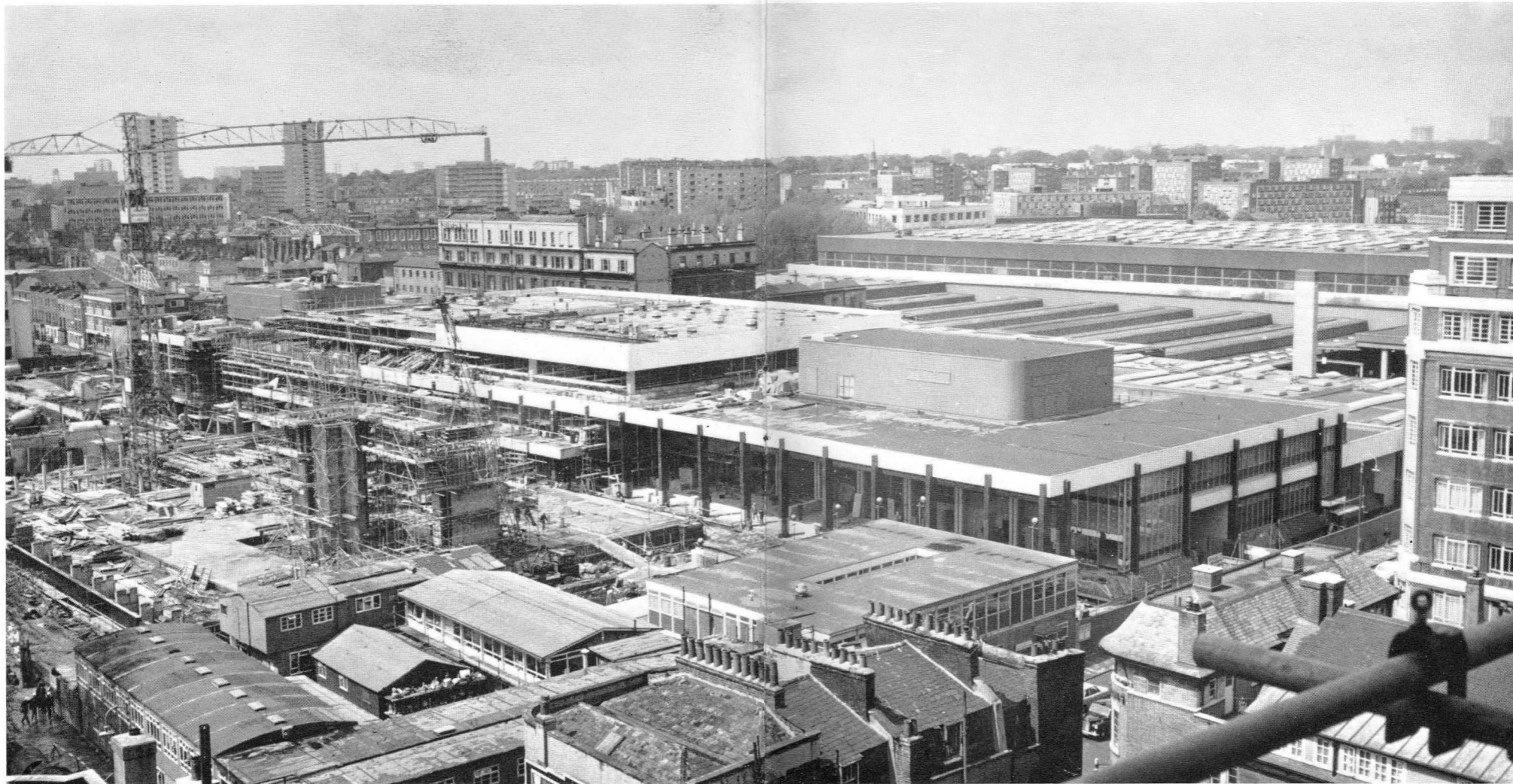
Nearing completion: panoramic view of Station with East Colnade on right
