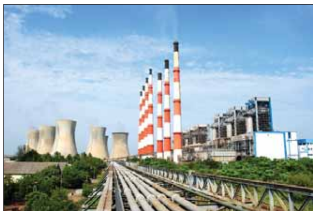
Thermal Power Plant of Neyveli Lignite Corporation, Neyveli, Tamilnadu
