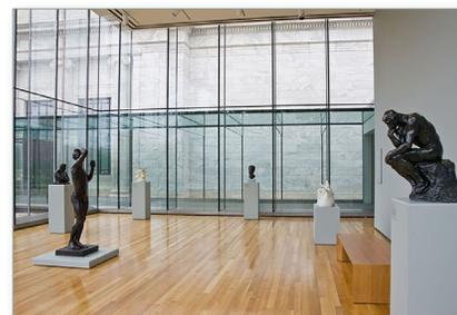
Phase 1 featured the installation of an innovative, 22-foot high, "double skin" glass-box gallery assembled utilizing no metal fastening.
