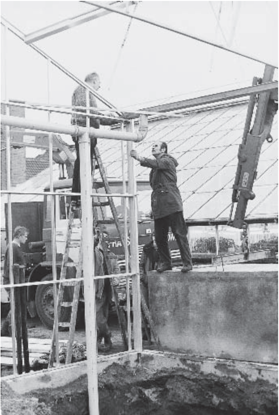
Building of new glasshouses, c. 1958. Archives of the wcs, Haarlem
