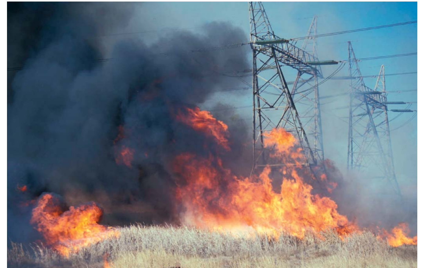
A grass fire burning underneath an Eskom transmission line
