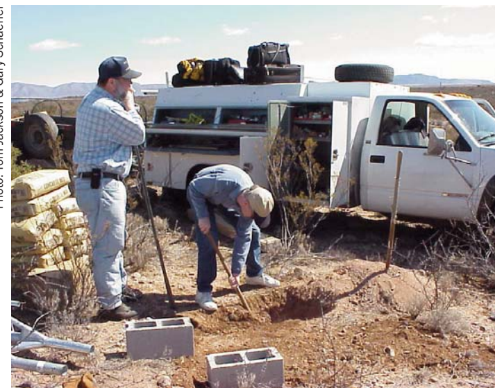
Installation of SCAN station in Arizona
