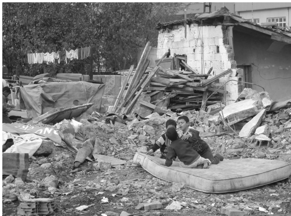
The demolitions in Sulukule / İstanbul, October 2006
