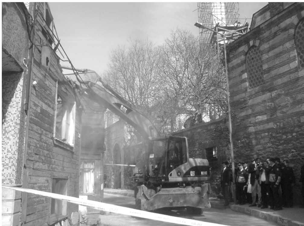
The demolition of a historical wooden house in Sulukule, October 2006
