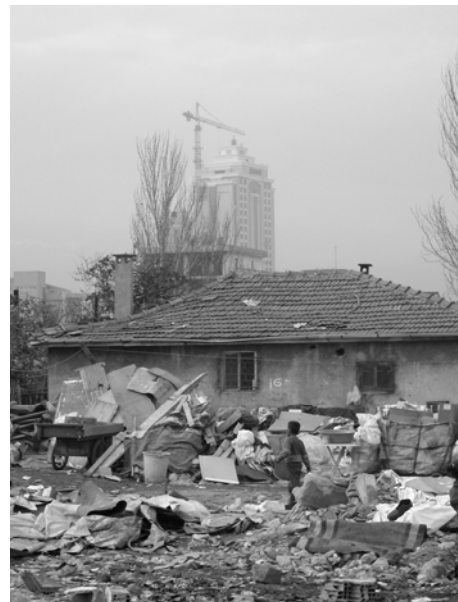
The demolitions in Küçükbakkalköy / İstanbul, September 2006
