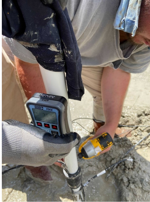
Figure 5-7: Handheld pretension of strain cable during Phase I installation
