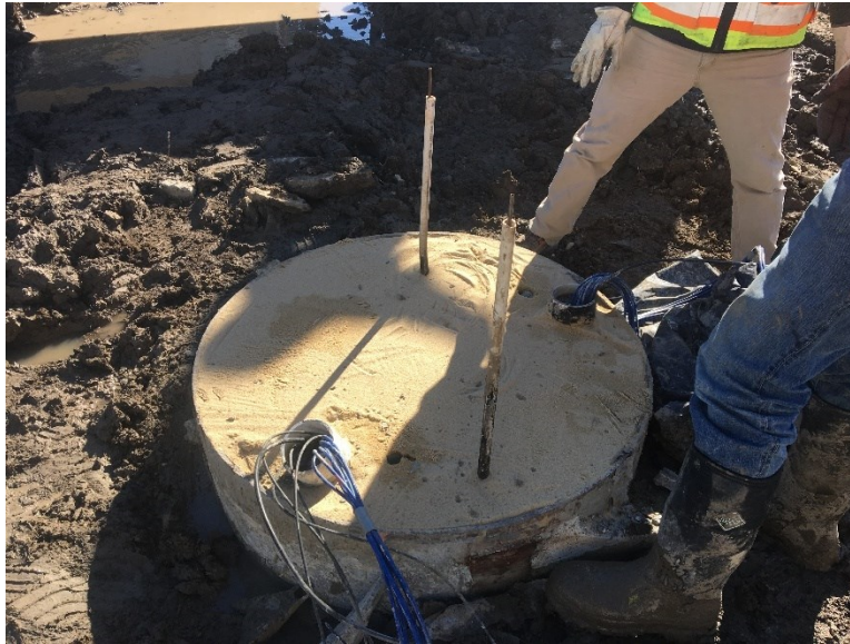
Figure 4-195: Sand bed preparation of test pile prior to load test
