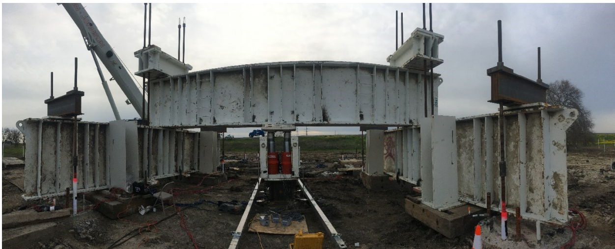
Figure 4-13: Load test frame
