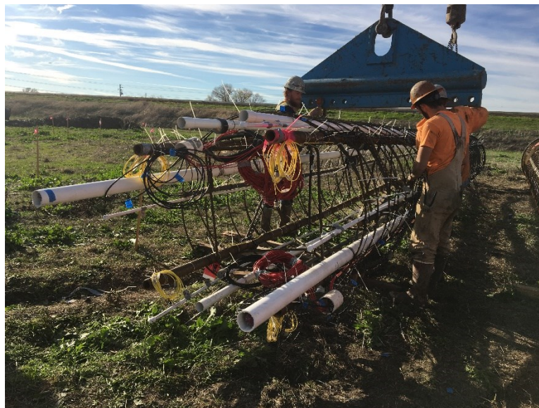
Figure 4-18: All instrumentation wiring installed and coiled; cage prepared for final pick
