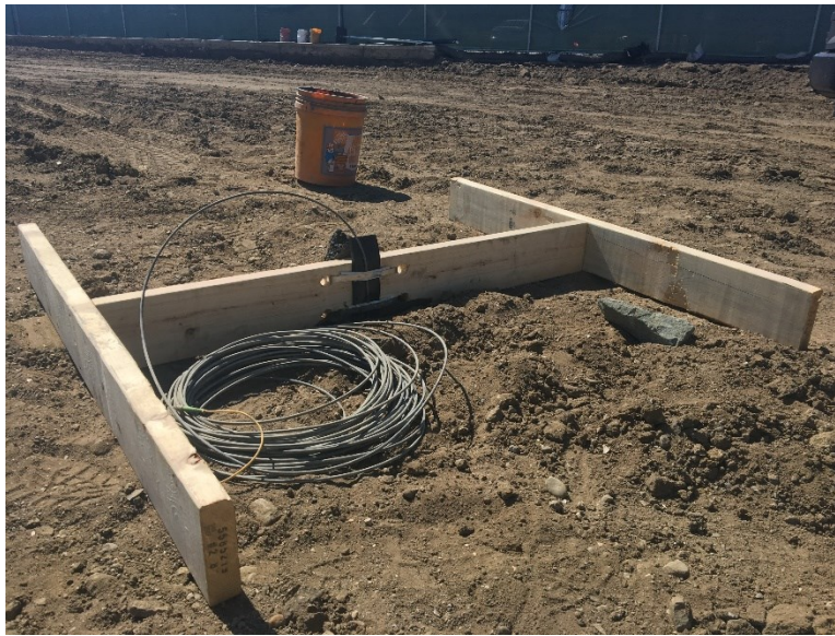
Figure 5-33: Completed fiber optic installation and tension frame, immediately following installation
