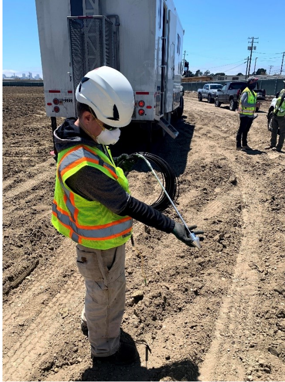
Figure 5-31: Prepared fiber optic cable and dummy CPT tip
