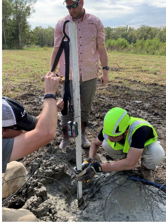
Figure 5-8: Ratchet-controlled pretension setup for strain cable during Phase II installation
