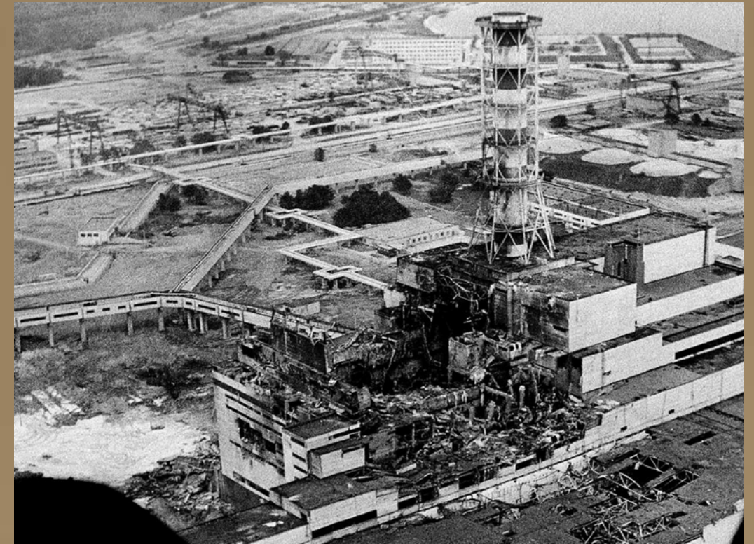
Image 2 The Chernobyl Plant explosion released around 40 GJ of energy -- equivalent to about 10 tons of TNT (Dubasov & Pakhomov, 2009).
