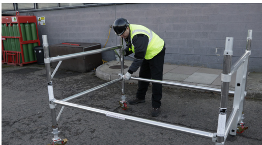
5. Fit another horizontal brace on the ladder side of the frames face down onto the 1st rung. Note: when standing inside the frames looking at the ladder frame, the ladder should be to the left hand side.
