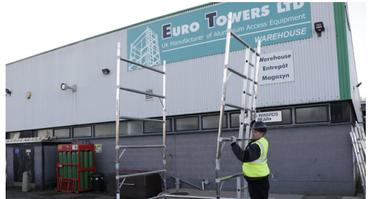
6. Fit the next set of frames onto the base, ladder frames run continuously up the left hand side. Note: see kitting page for frame lists.
