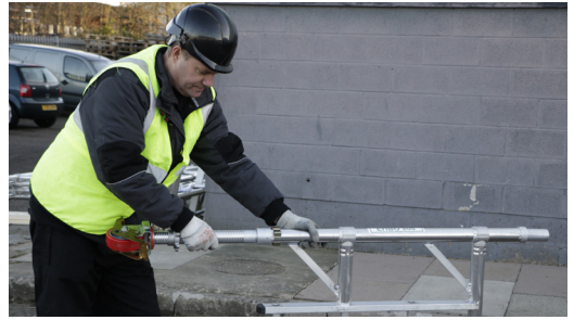
2. Insert the castors into the adjustable legs. Insert 2 legs and castors into each 2 rung frame.
