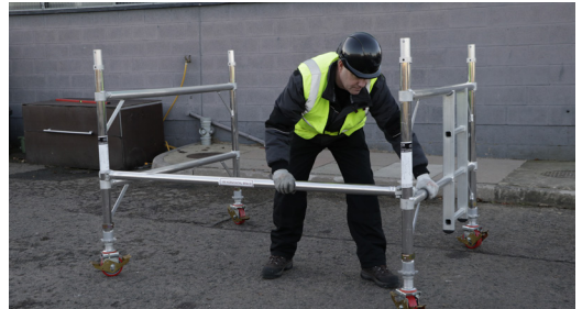
4. Fit one horizontal brace on the plain side of the frames to the vertical of the frames above the 1st rung connecting the 2 frames together. (Integral ladder must be on the left hand side)
