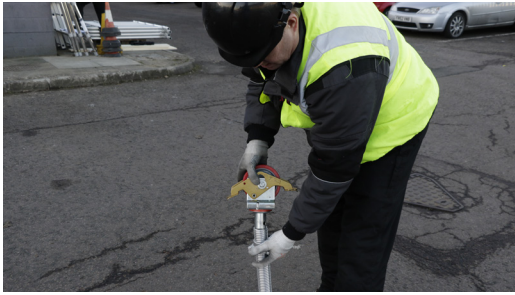
1. Insert castor wheels into adjustable legs
