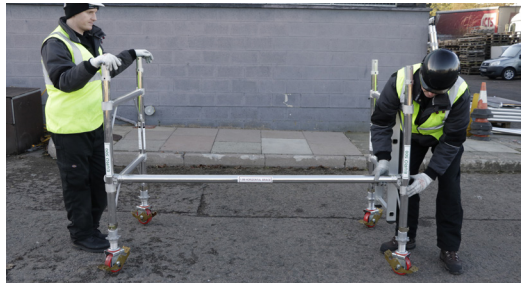
4. Fit one horizontal brace on the plain side of the frames to the vertical of the frames above the 1st rung connecting the 2 frames together.
