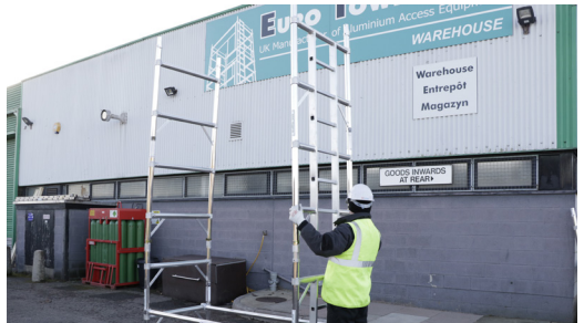
5. Fit the next set of frames onto the base, ladder frames run continuously. Note: see kitting page for frame lists.
