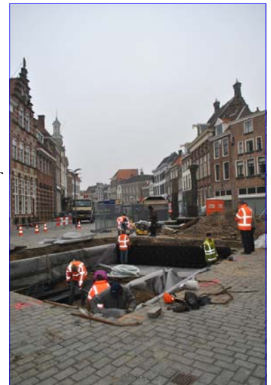
Fig. 3. General view of one of two planting holes for trees within the old city of Zutphen. Photo from ref. 1.
