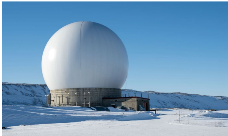
A radar dome belonging to the 23 rd Space Operations Squadron Detachment 1 at Pituffik Space Base, Greenland on April 4, 2023. The detachment’s extreme northern location allows contact with polar orbiting satellites 10-12 times per day. (U.S. Space Force photo by SrA Kaitlin Castillo)
