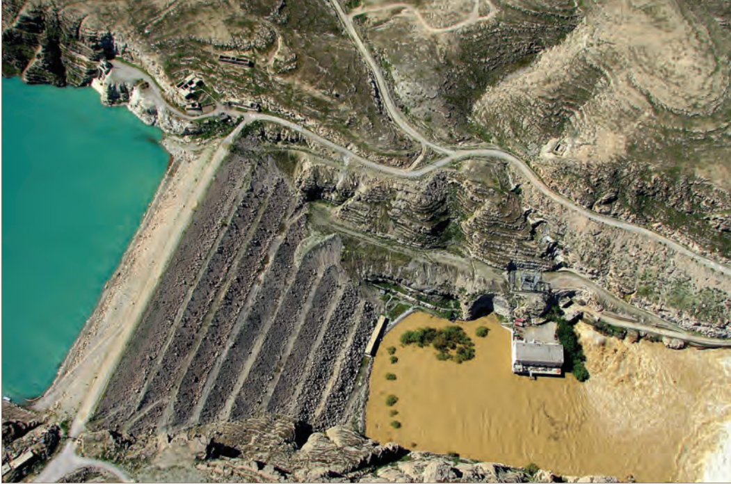
An aerial view of the Kajaki Dam in Helmand Province, a key part of the Kandahar Helmand Power Project. (USAID photo)
