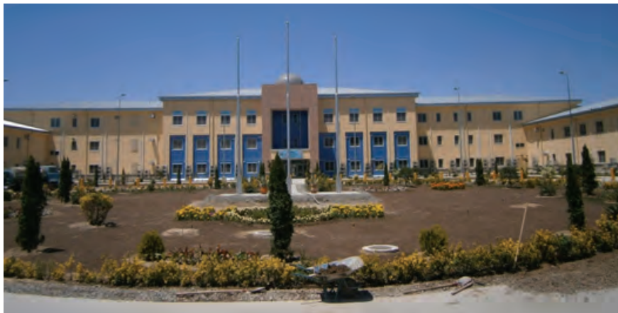
Newly inaugurated MOI Headquarters building in Kabul. (CSTC-A file photo)
