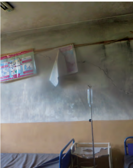
SIGAR's site inspections of health facilities in Kabul revealed basic structural concerns at most facilities, such as cracked walls. (SIGAR photo)
