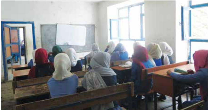
Broken windows and doors at a USAID-funded girls' high school in Bamyan Province. (SIGAR photo)
