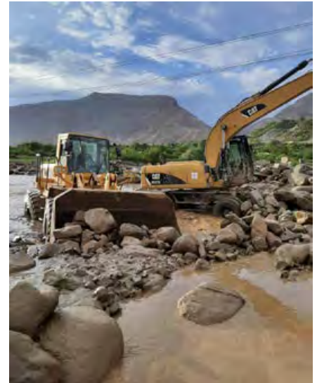
Construction crews work to clear the Parwan-Bamyan road after August flooding. (Taliban regime photo)
