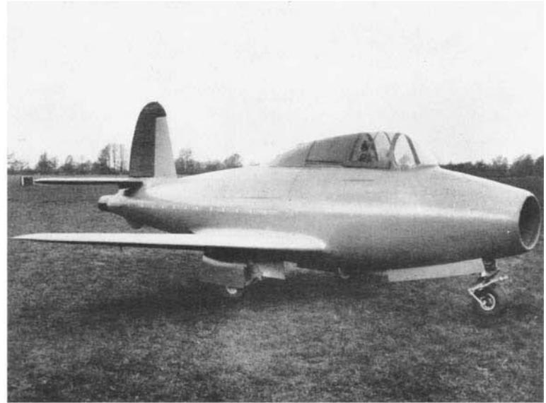
Fig. 41. The Gloster-Whittle Experimental Aeroplane E28/39
